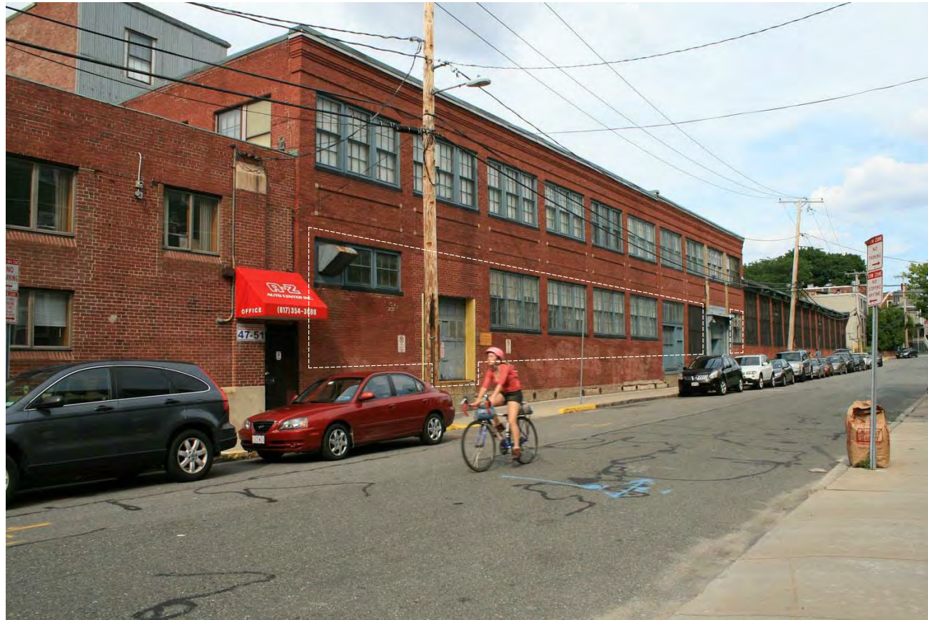
The two story section of the building has been modified over time and will receive modifications to enable residential use.
