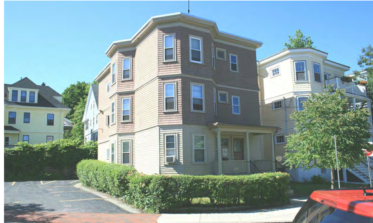
General Residential Context Across the Street from Building
