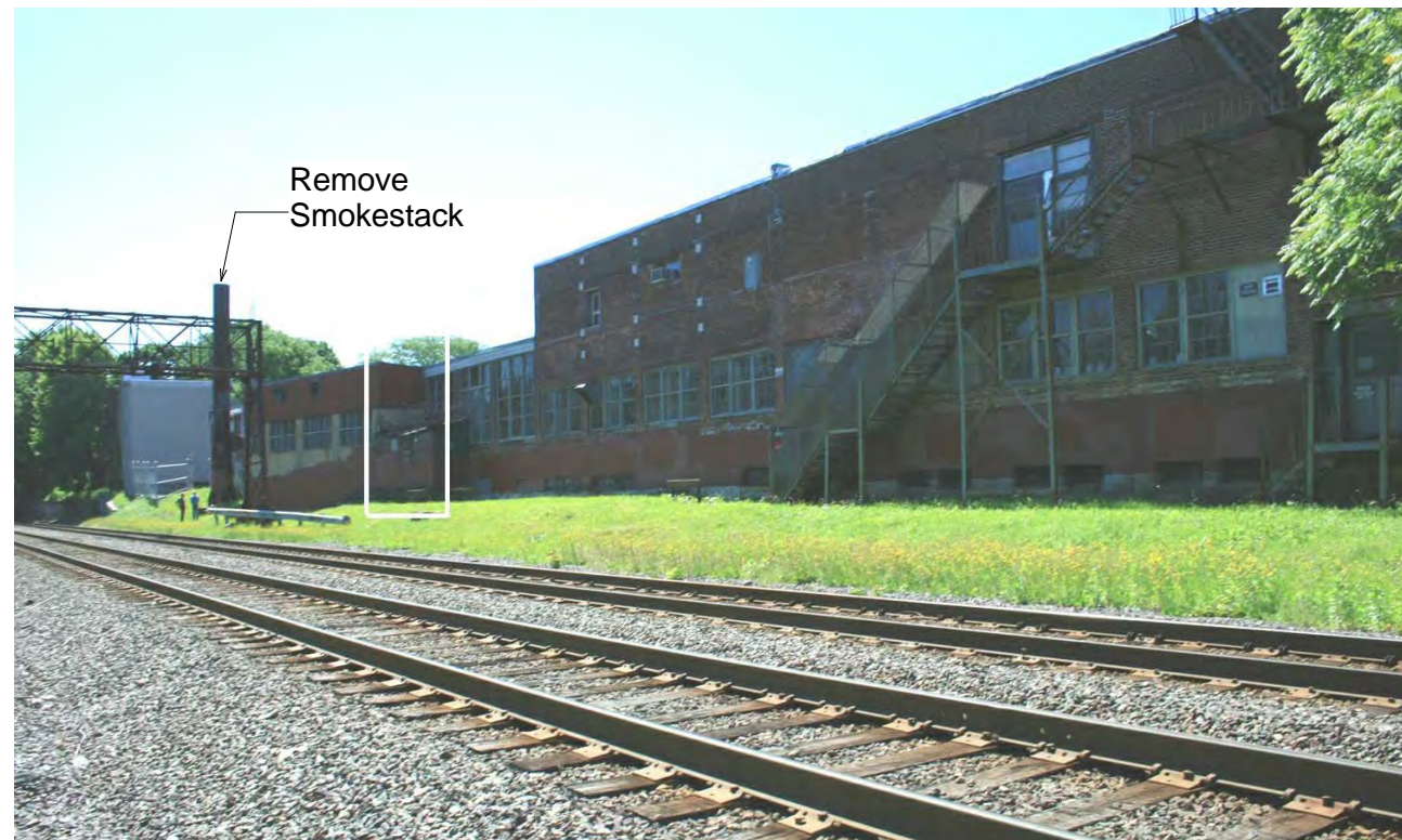
Existing building looking east on rail road right-of-way. New windows will replace brick infills. The storage shed addition will be removed.
