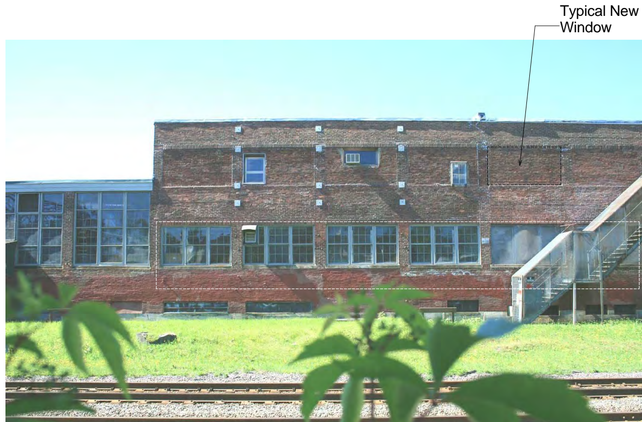
Rear side of existing building showing areas of facade failure. Existing window openings were bricked in. Bricks will be removed and new windows installed.
