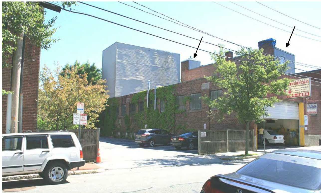
Property to the East of Existing Building (45 Richdale) and Existing Third Floor and Elevator Penthouse Structure.
