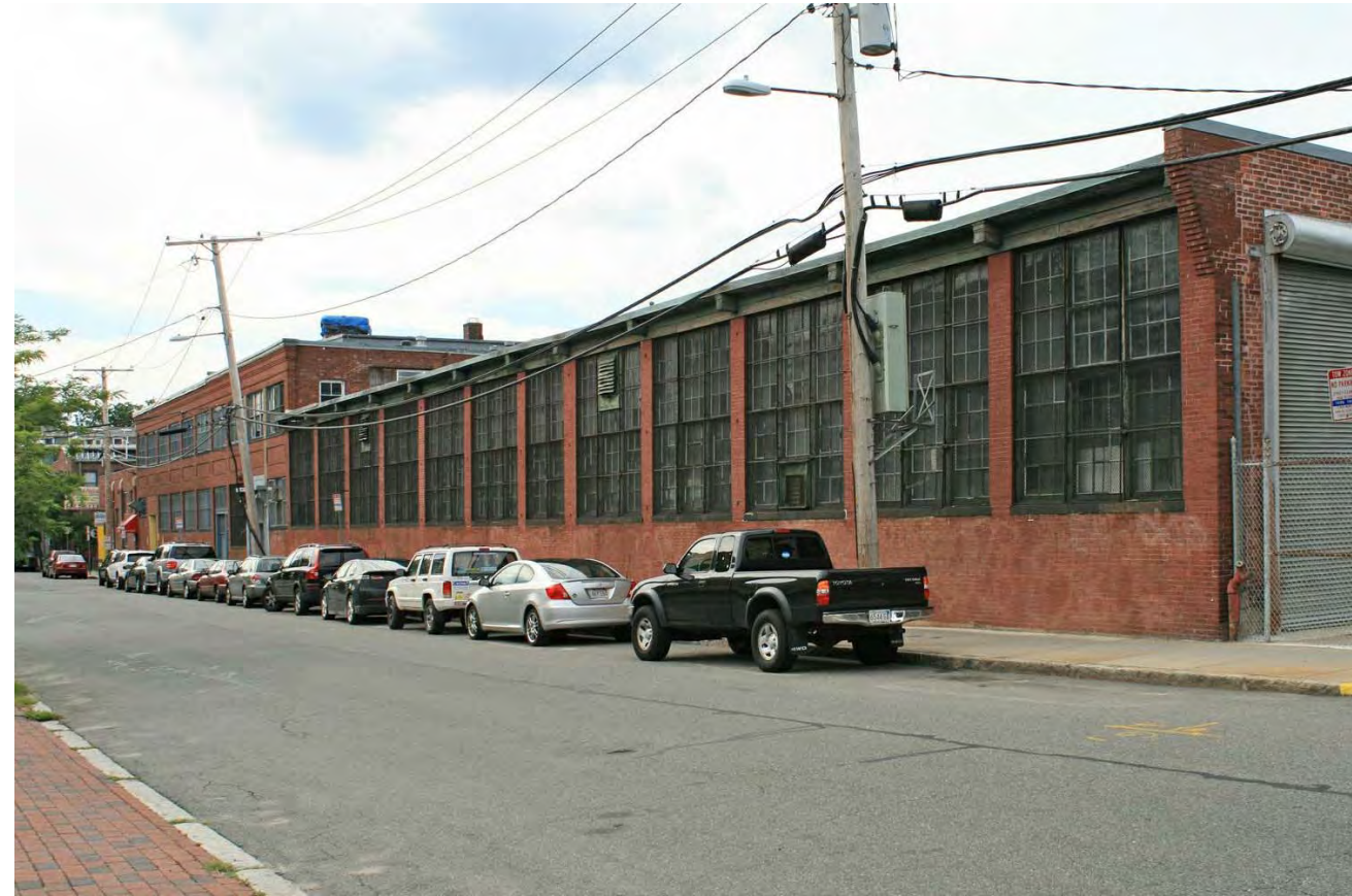
The one story section of the building.
