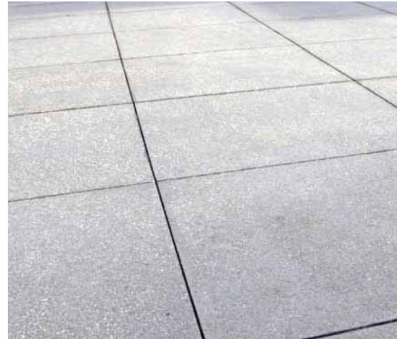
VEHICULAR DRIVEWAY PAVING - CAST IN PLACE CONCRETE
