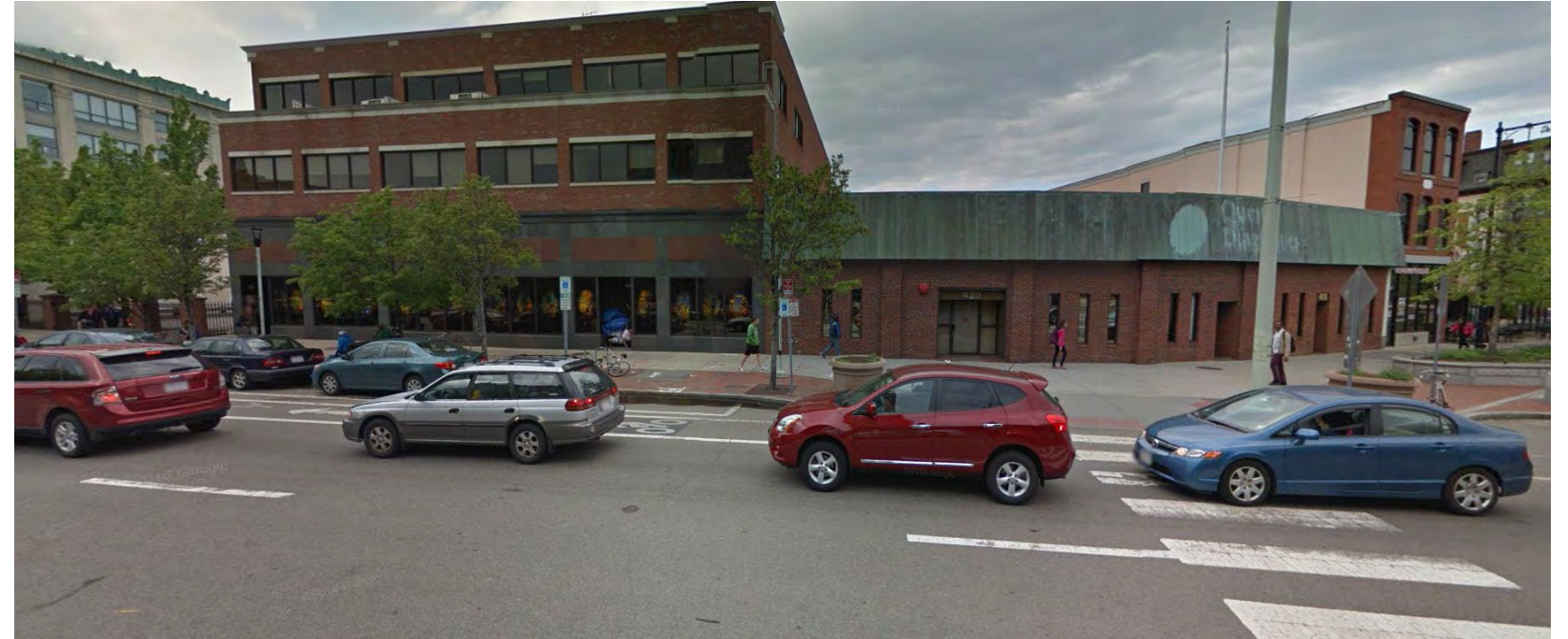
Project Site frontage along Massachusetts Avenue
