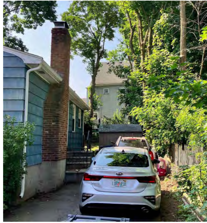
EXISTING ENTRY, WEST ELEVATION
