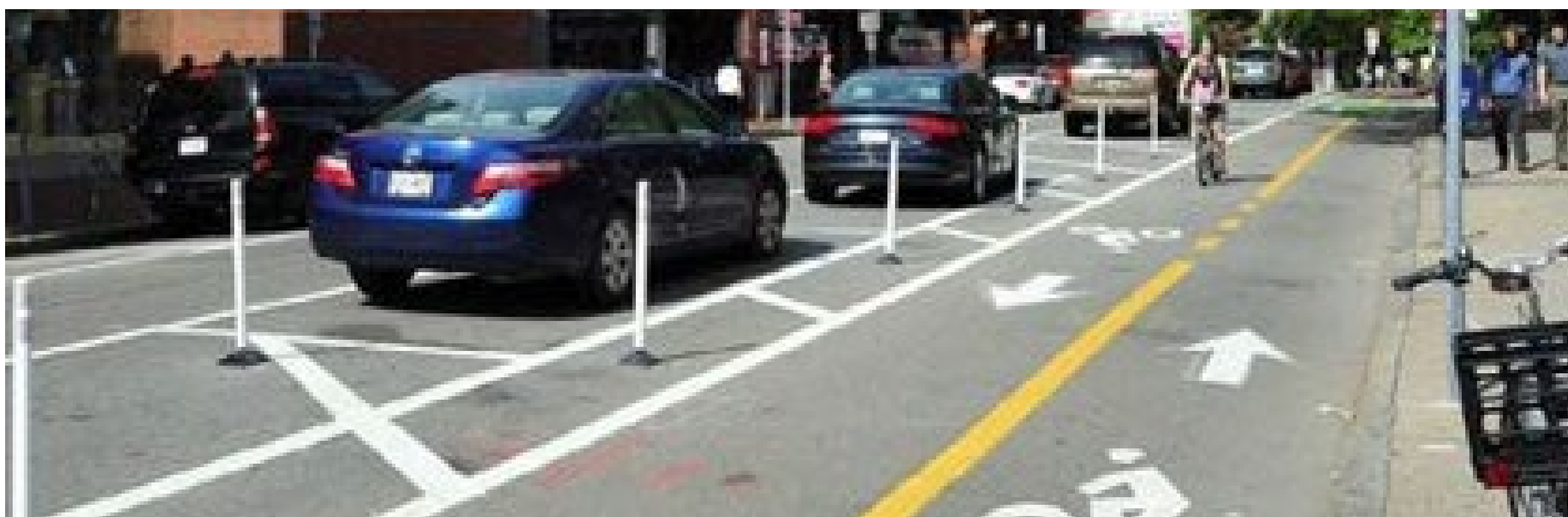
A separated bike lane on Brattle Street
