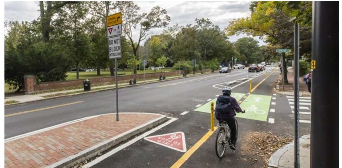
Idea 2: Corner treatments to better protect people walking and biking and slow turning drivers at unsignalized locations
