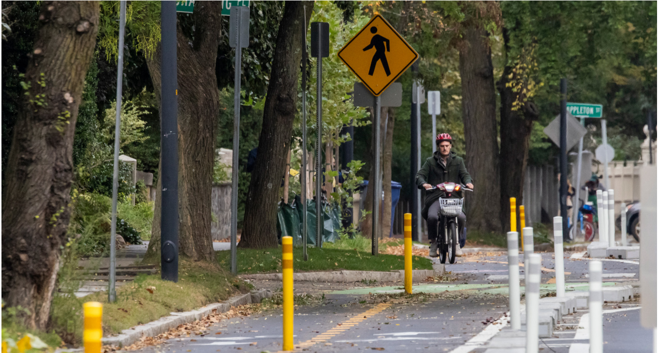
Brattle Street Safety Improvement Project, October 2023 by Kyle Klein.
