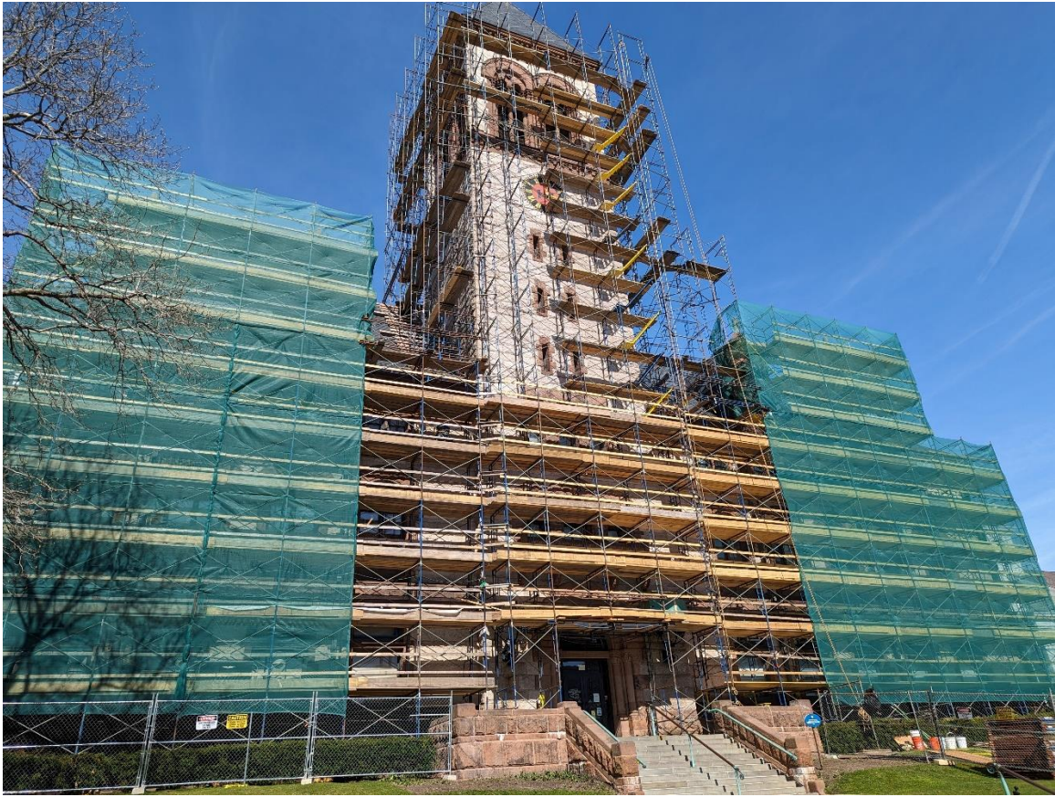
City Hall facade repairs
