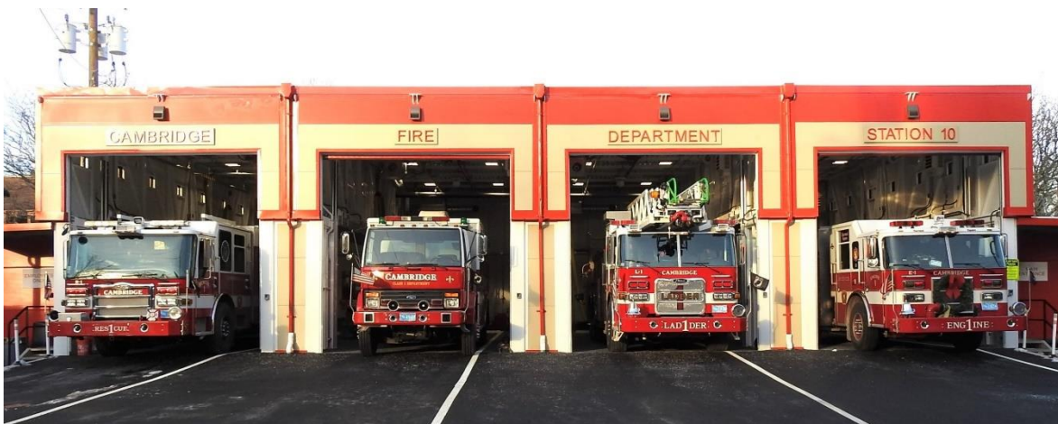
Temporary location of Engine One and Ladder One during Headquarters renovation
