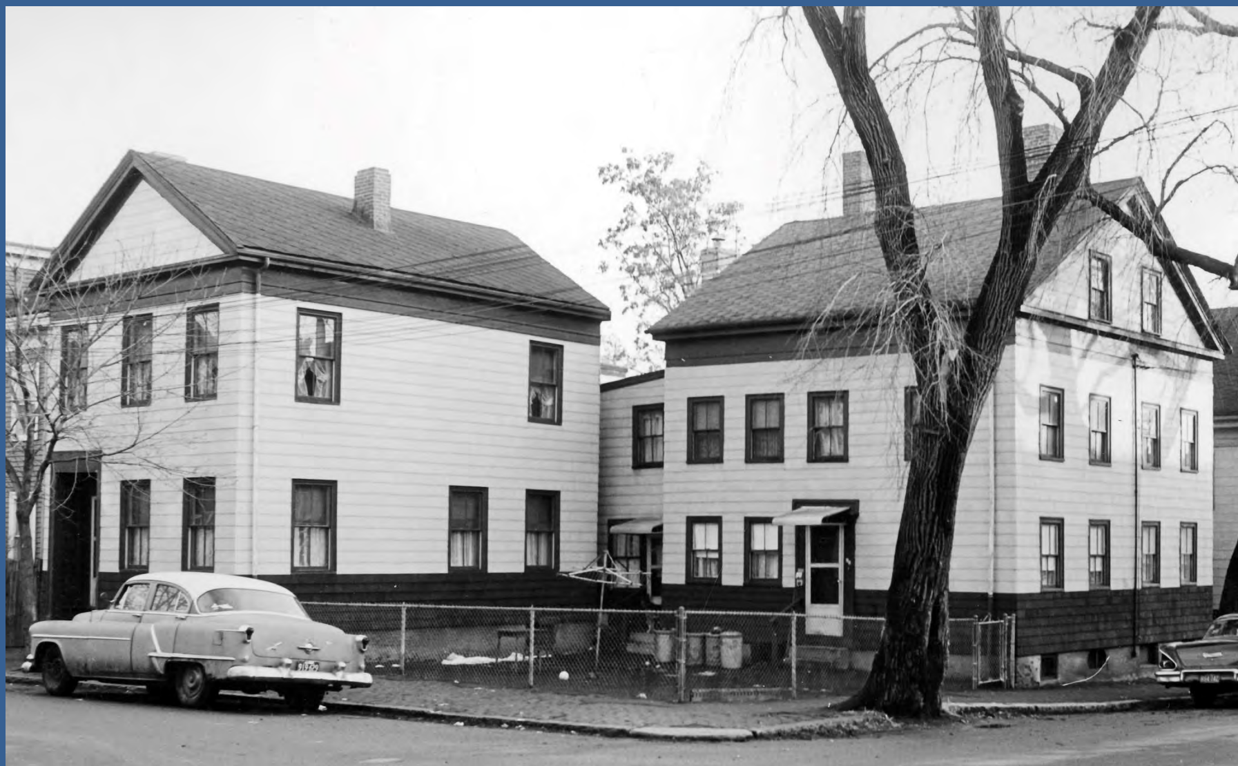
James Smith House, 98-100 Sciarappa Street (1843)
