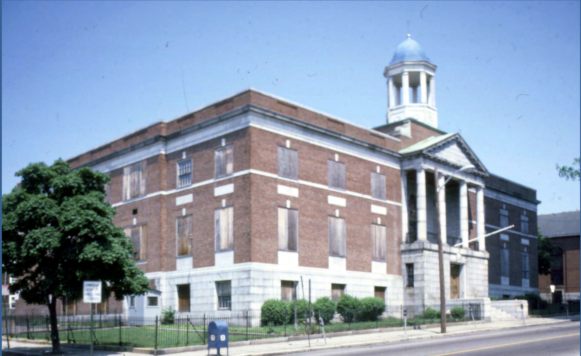
Boarded up and vacant, 1972- (Photo 1984)
