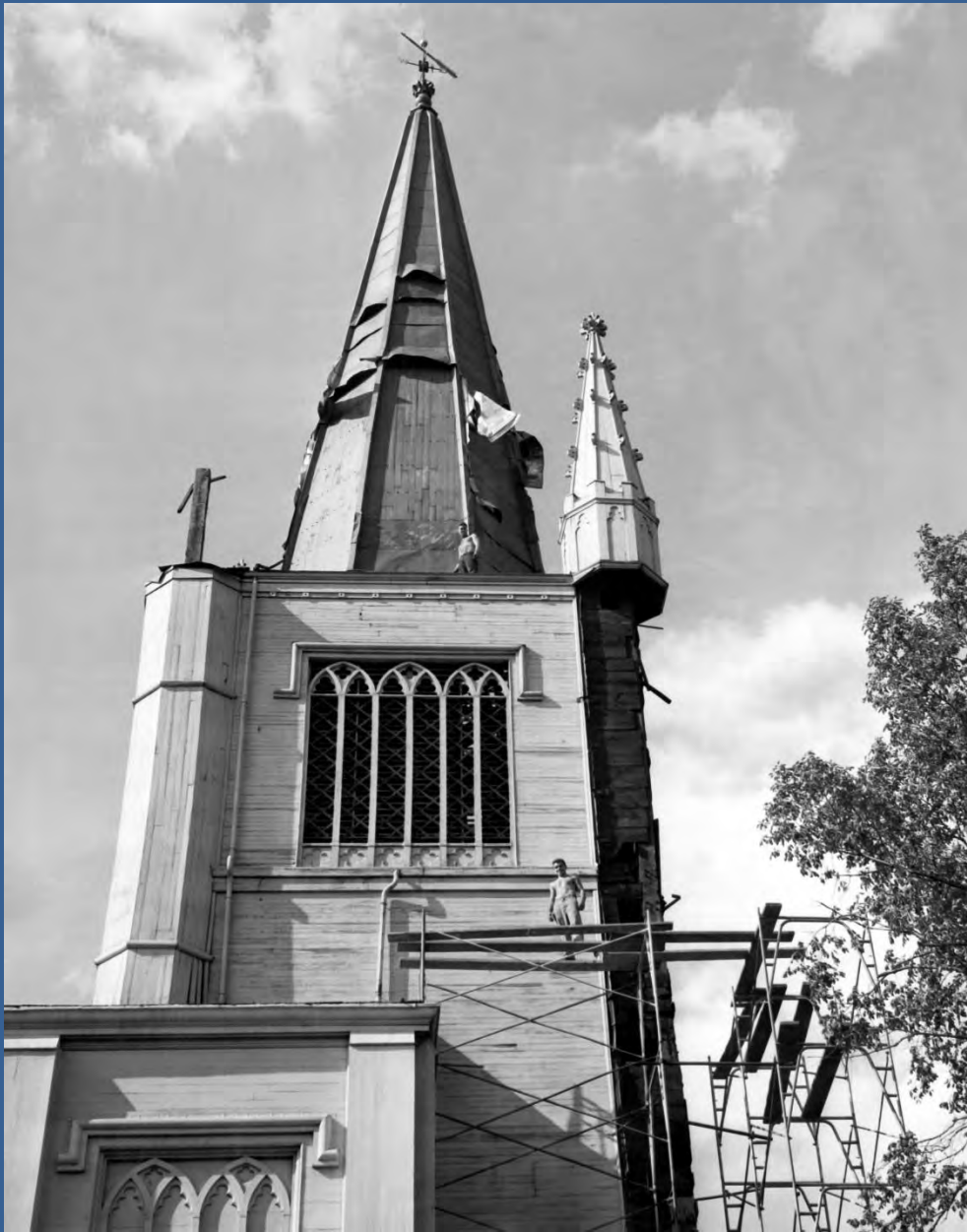
Removal of decorative elements weakened by hurricanes in 1954.
