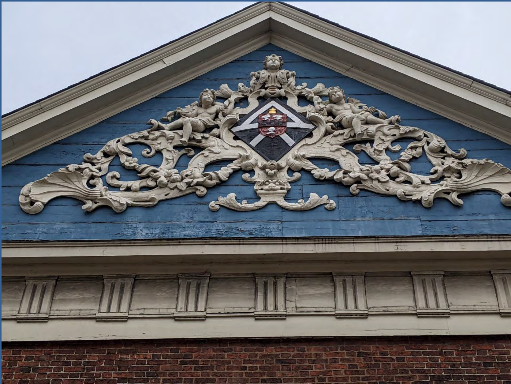
Original crest of the Holden family, west facade
