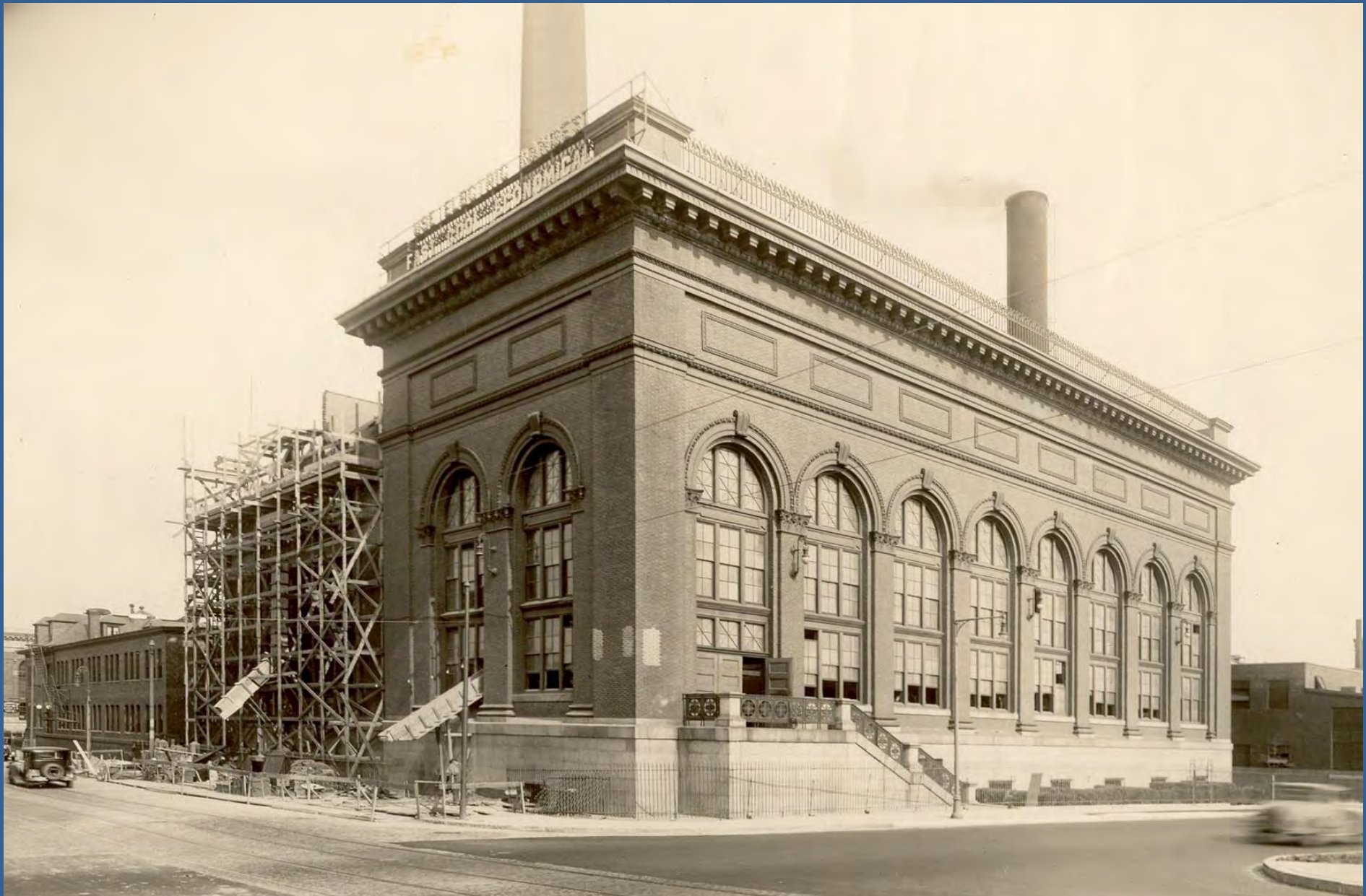
Cambridge Electric Light Co. Blackstone Station (1901, Sheaff & Jaastad, architects). Photo 1918
