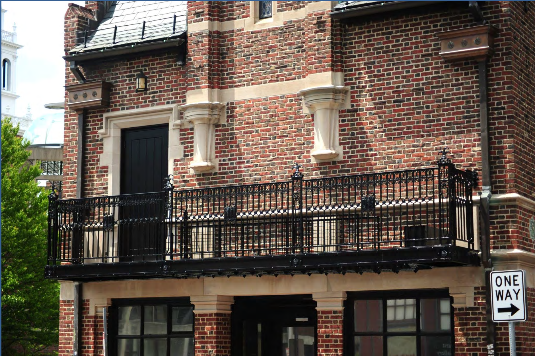
Egress door and fire escape, 2014
