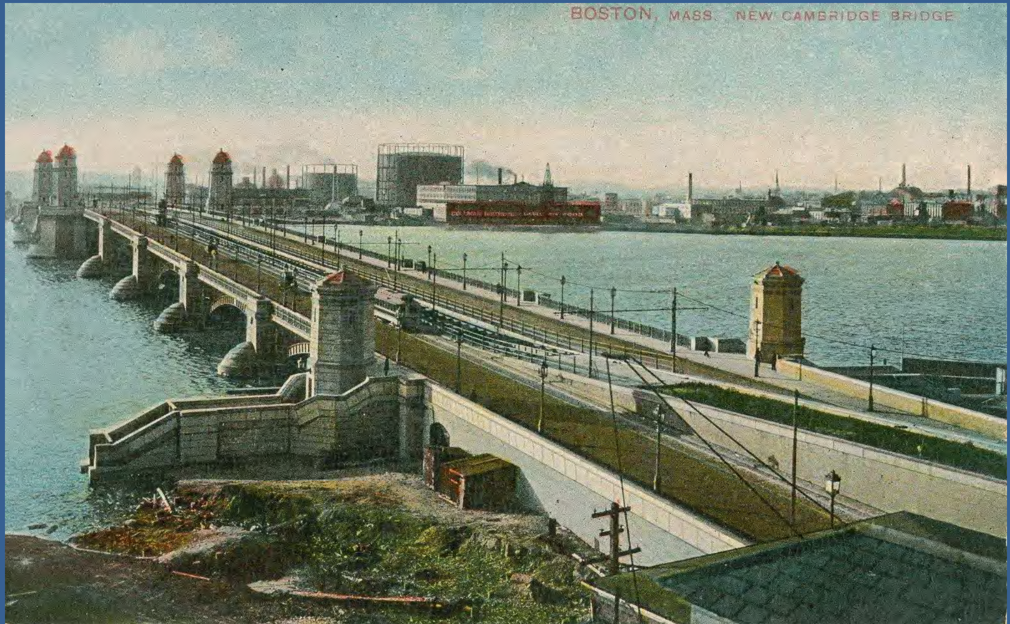
Longfellow Bridge (1900, Edmund Wheelwright, consulting architect)
