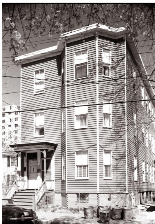
54-56 Banks Street, CHC survey image, 1965.
