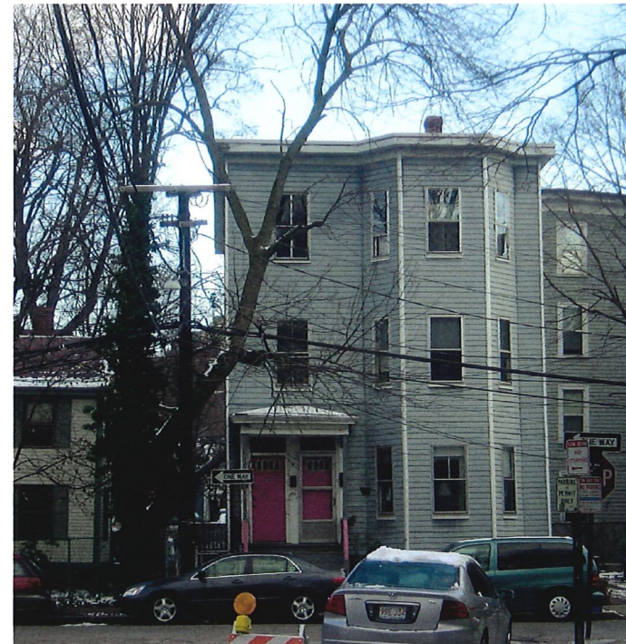
Pre-Renovation Condition: West Elevation
