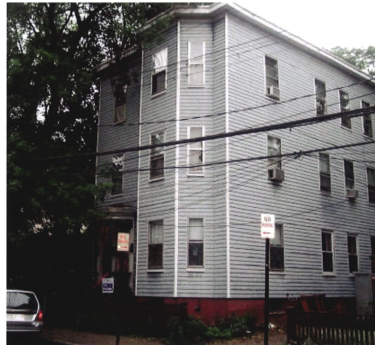
Pre-Renovation Condition: West Elevation
