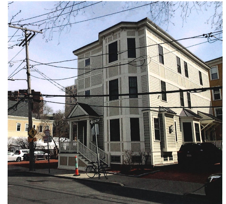
Current Condition: South / West Elevation
