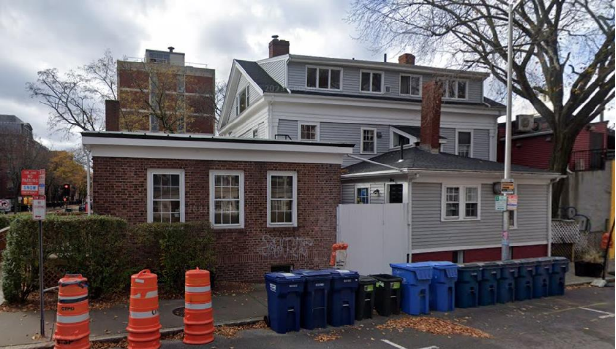
Rear elevation, 43-45 Mt. Auburn Street
