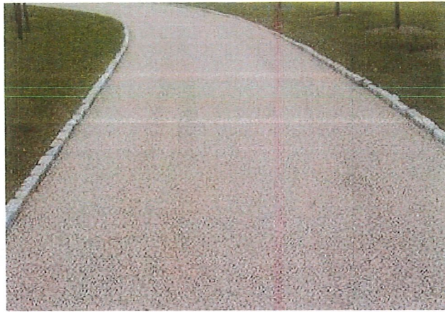
E Chip-Seal Finish at Asphalt Driveway L-3
