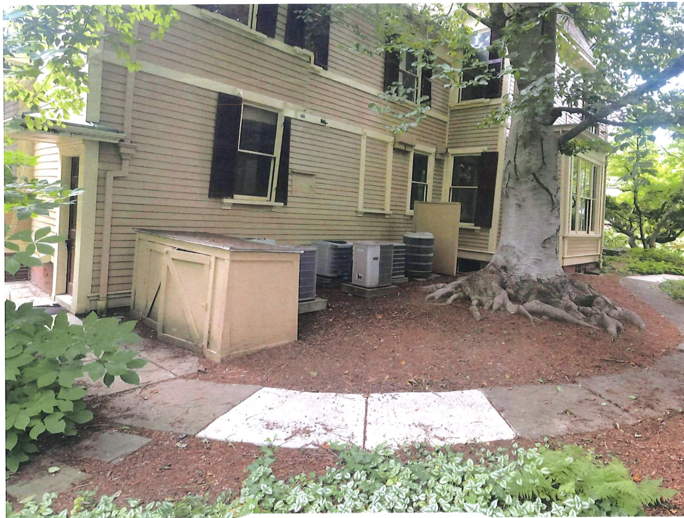
B Existing Utilities and Beech Tree behind the House L-9
