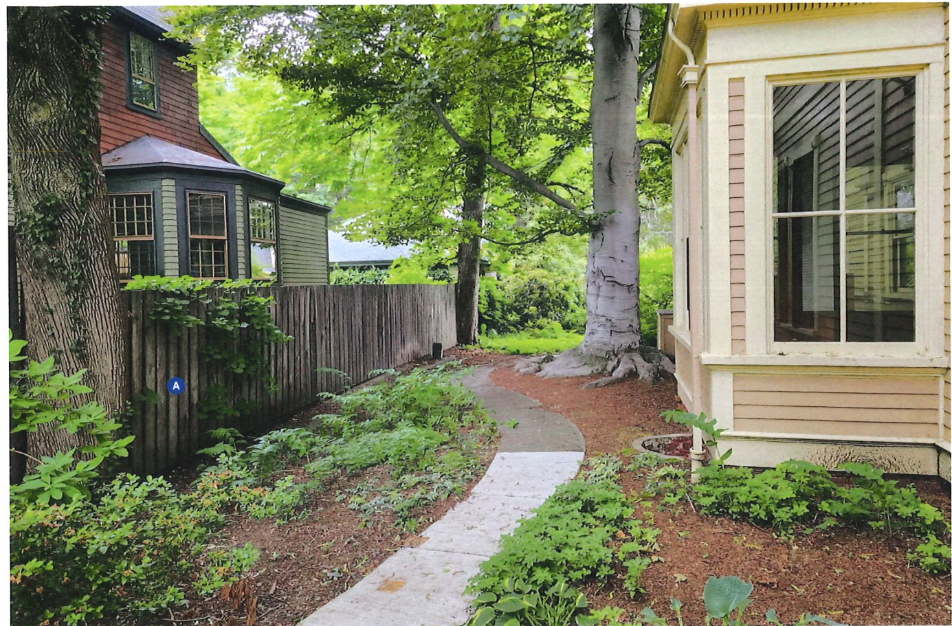
Key: A The top of the new fence shall slope with the grade to match the existing condition
