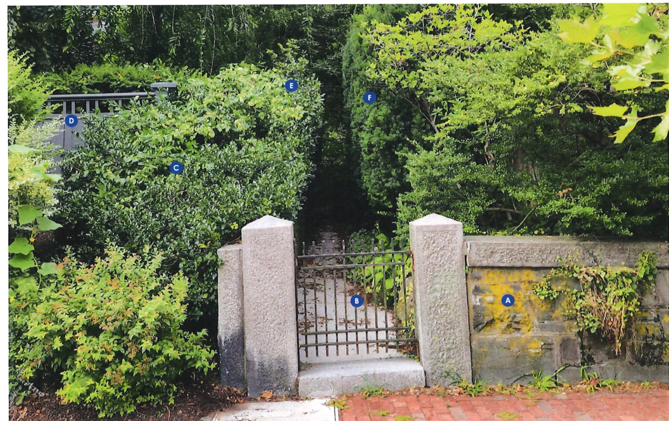
Key: A Existing 40"ht. stone wall to remain. B Existing 36" ht. pedestrian gate to be replaced. C Existing Holly to remain D Existing fence on abutter's property to remain E & F Existing Yew to remain
