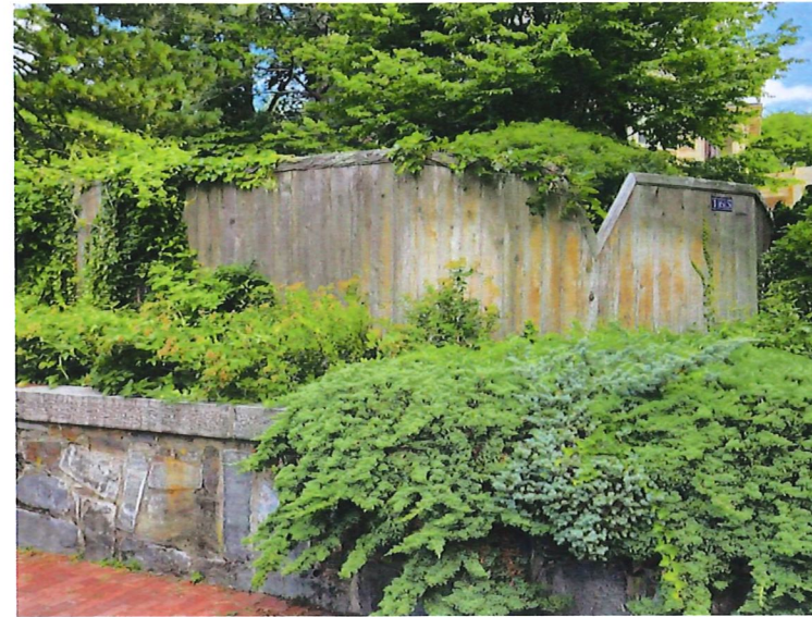
D 5' ht. Existing Vertical Board Fence at Street L-5
