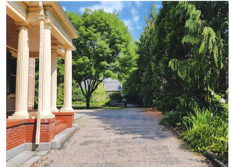
C View from Driveway within Property L-5
