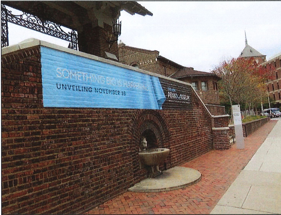
Image 7A (above): Penn Museum, University of Pennsylvania (3260 South Street, Philadelphia, PA) – Similar sign application from the same manufacturer on brick façade material. The property is listed on the City’s local historic register and notes an original construction date of 1899, a similar period to Knafel Center which was constructed in 1898. The sign was used to announce the reopening of the museum as part of their multi-million dollar building transformation project (November 2019).
