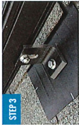
ATTACH L-FOOT TO RAIL
