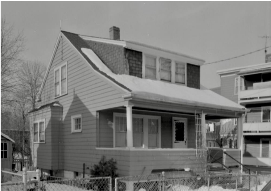
24 Newell Street before 1991 renovations. CHC Survey image 06-1972.
