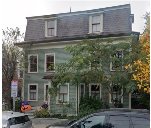
31-33 Willard Street, After (2020)
