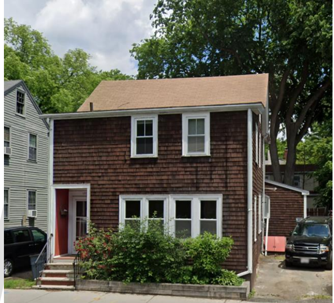
137 Mount Auburn Street, original structure (2016)
