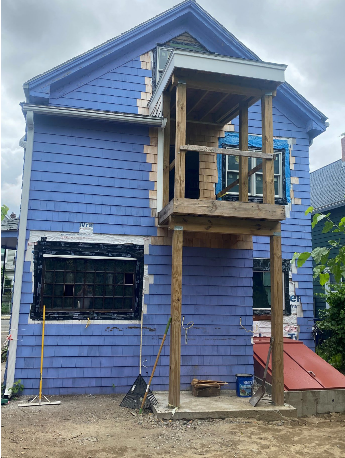
View from rear yard – East Facade
