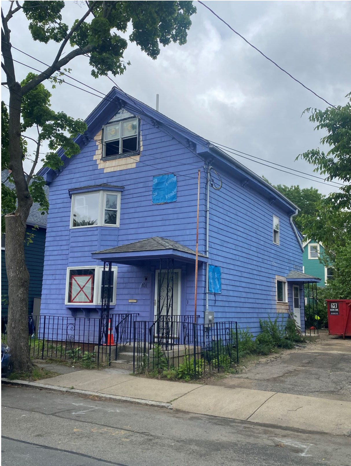
View from street – SW Corner at Driveway
