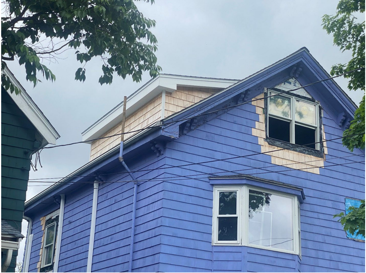
View from street – Shed Dormer @ North Façade
