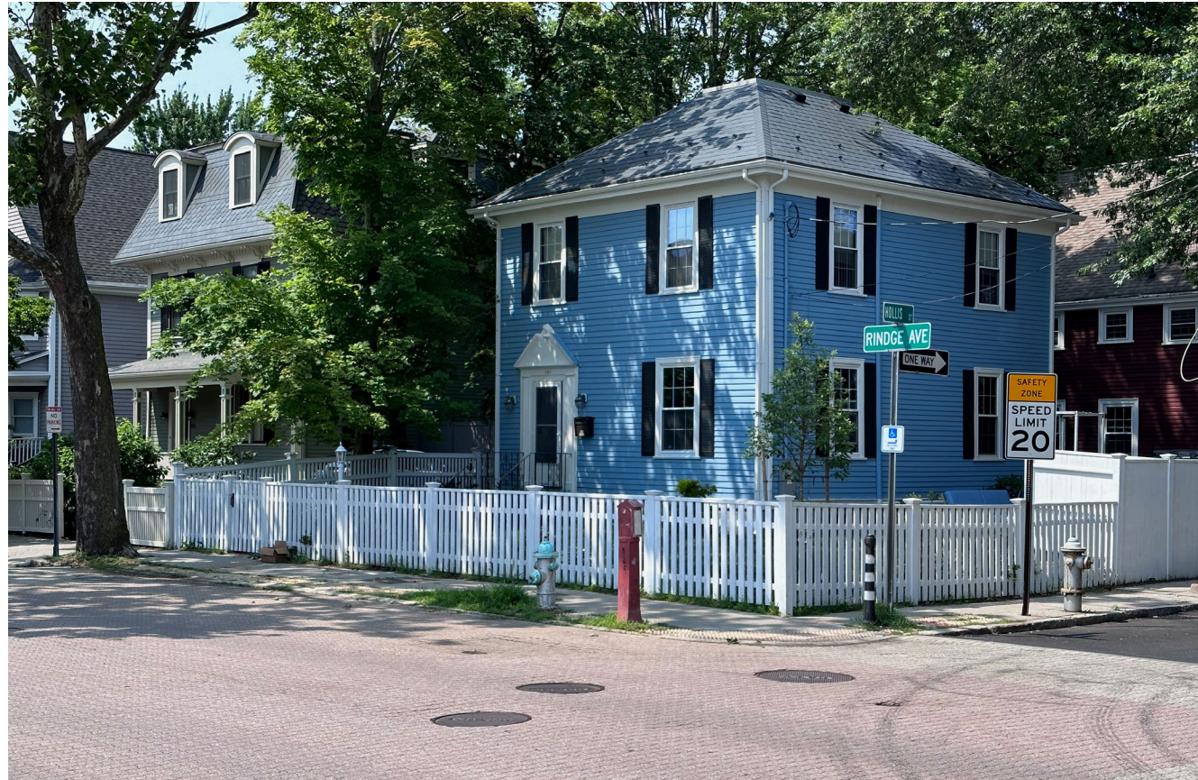
1.) 107 Rindge Avenue, front corner view
