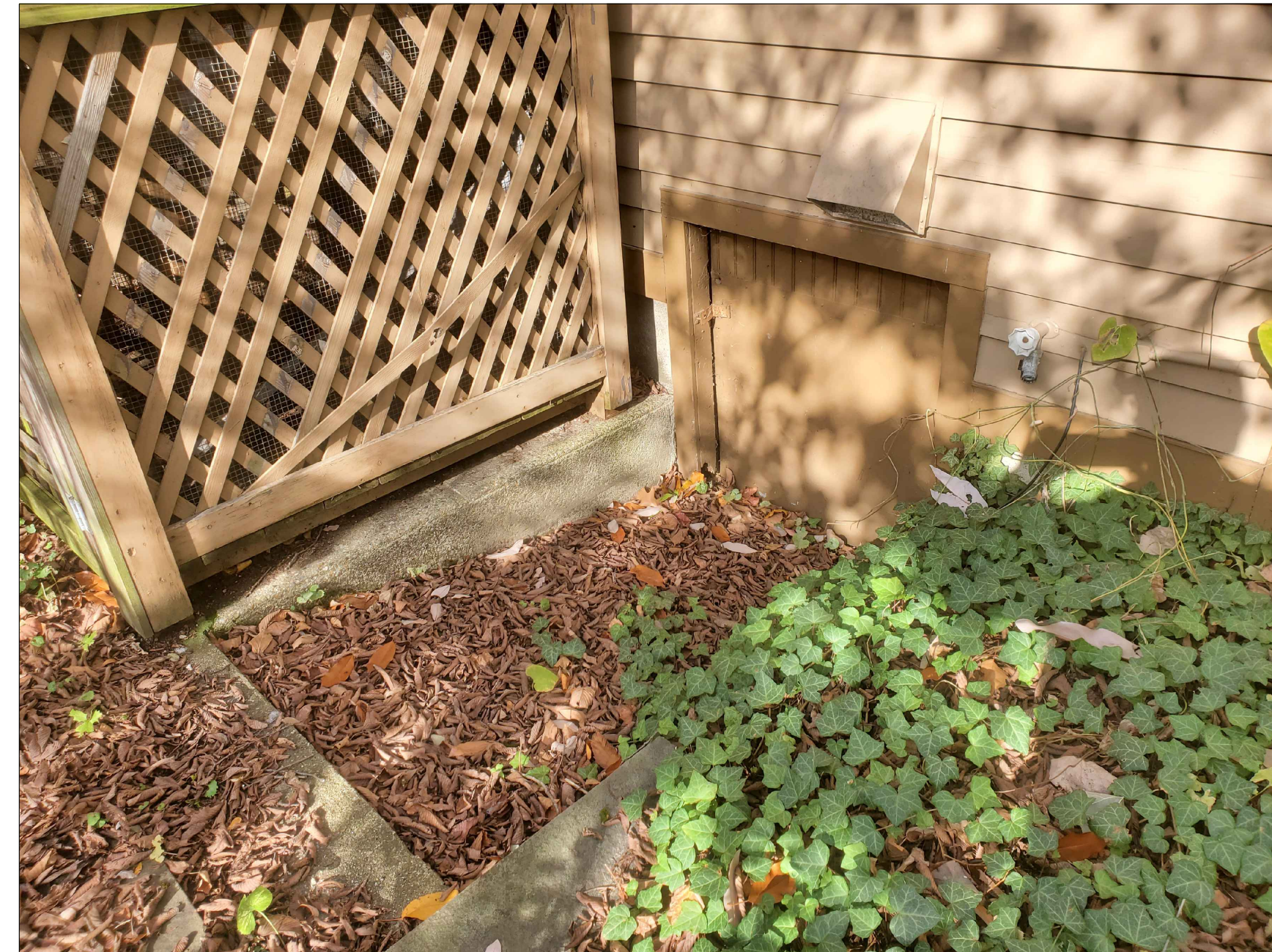
7 Stairs to Crawl Space at South Elevation
