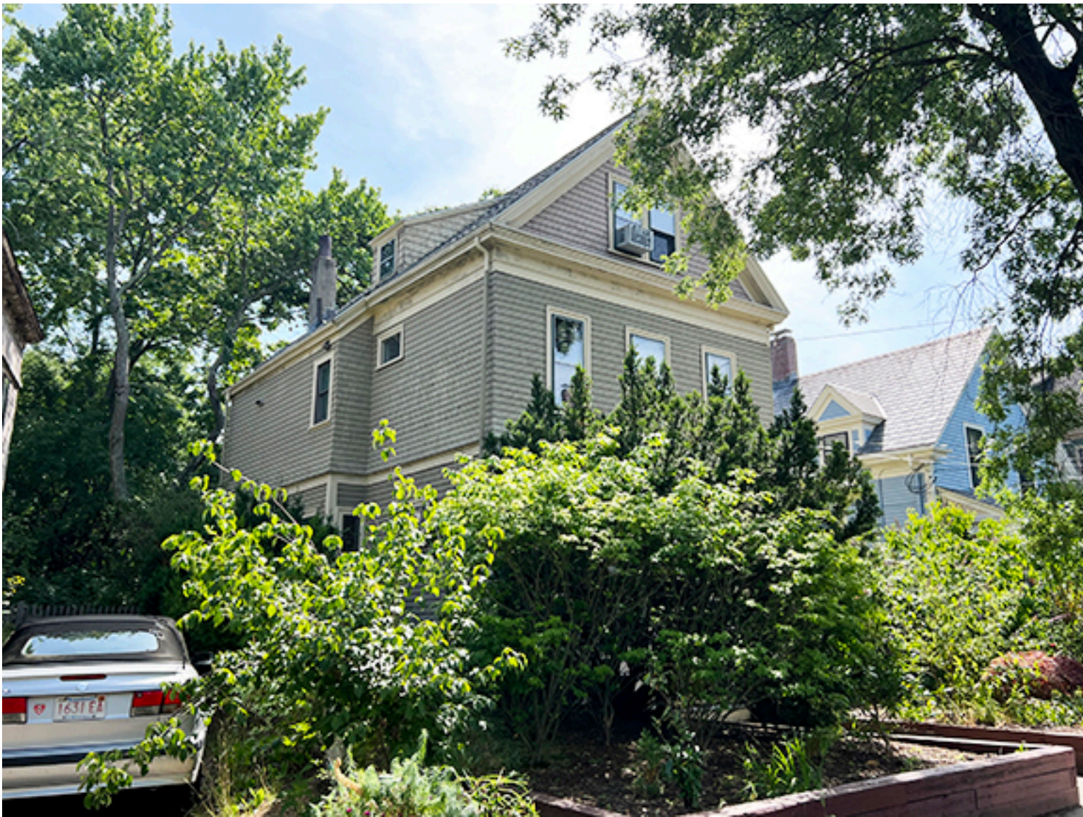
EXISTING STREET VIEW FROM LEFT
