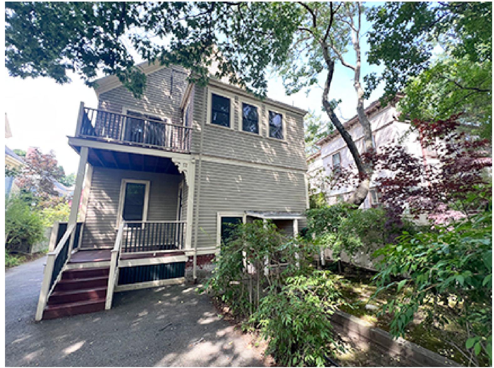
VIEW OF REAR
