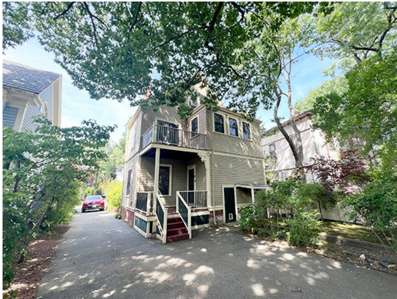
VIEW OF REAR
