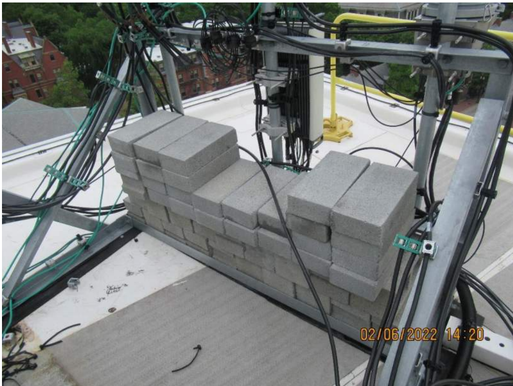
Photo 4: Sample photo illustrating an existing ballast tray at an existing antenna mount.
