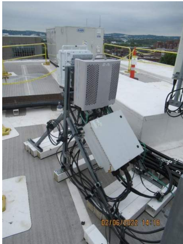
Photo 6: Sample photo illustrating an existing sleeper-style RRH ballast sled.
