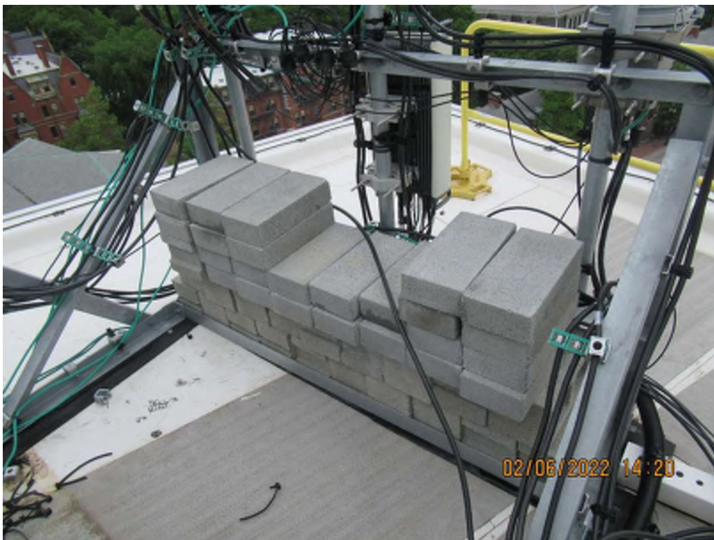
Photo 4: Sample photo illustrating an existing ballast tray at an existing antenna mount.
