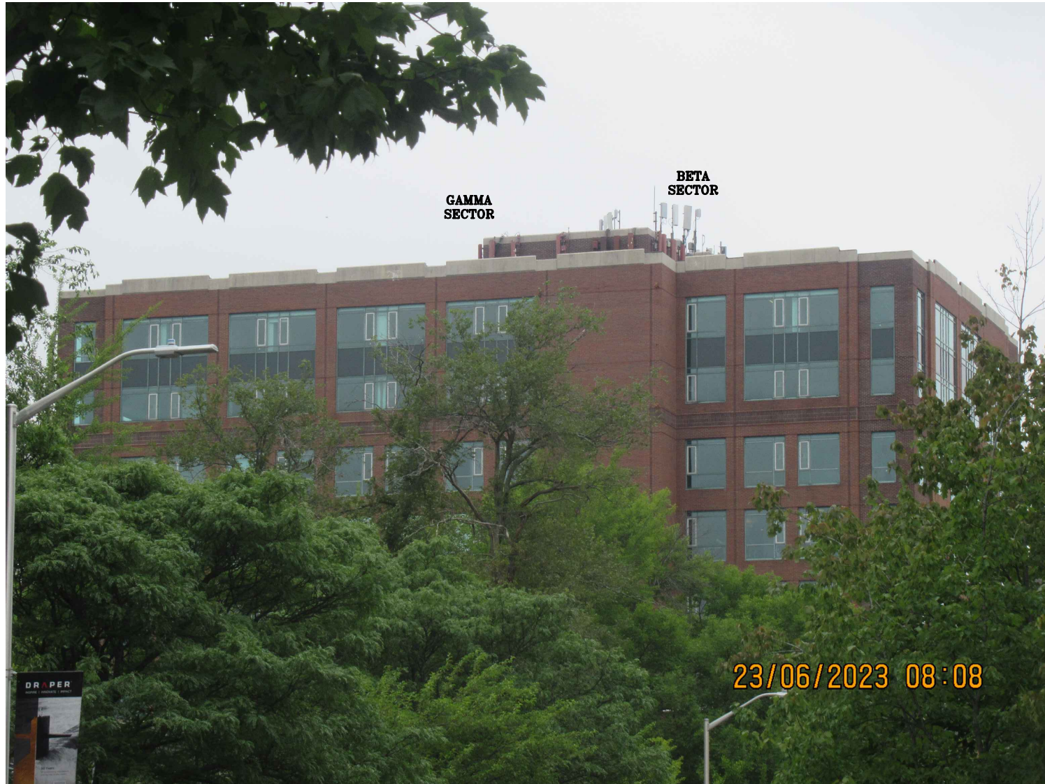
VIEW NORTH FROM PORTLAND ST
