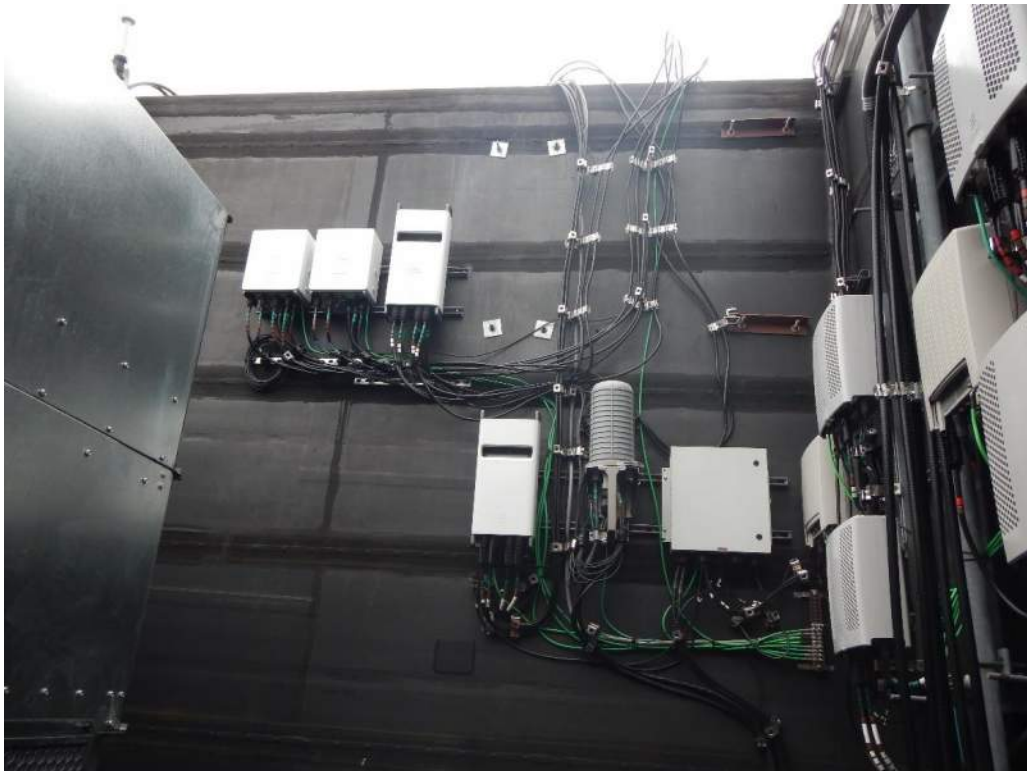
Photo 4: Sample photo illustrating the existing RRH's.
