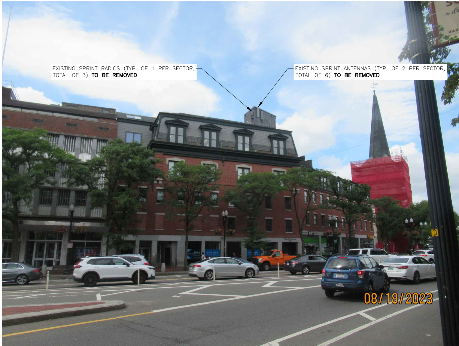
VIEW NORTHWEST FROM MASSACHUSETTS AVE
