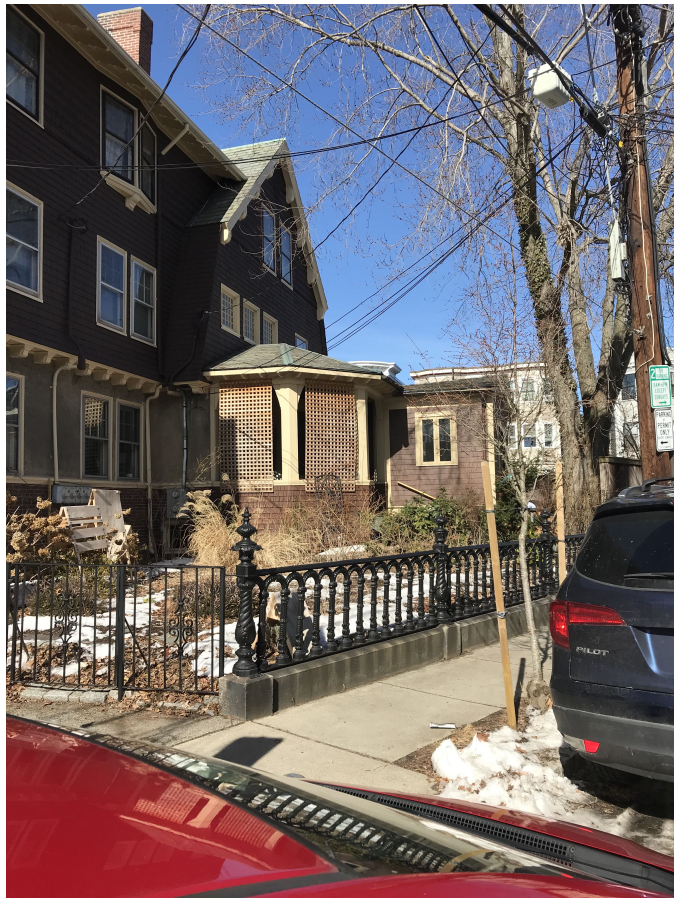
VIEW FROM FAYETTE STREET
