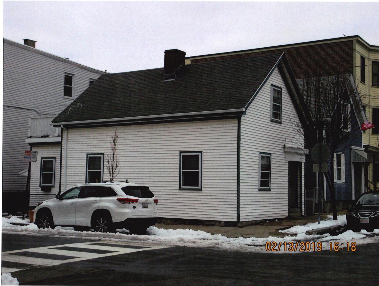
145 FIFTH STREET EXISTING STREET VIEW
