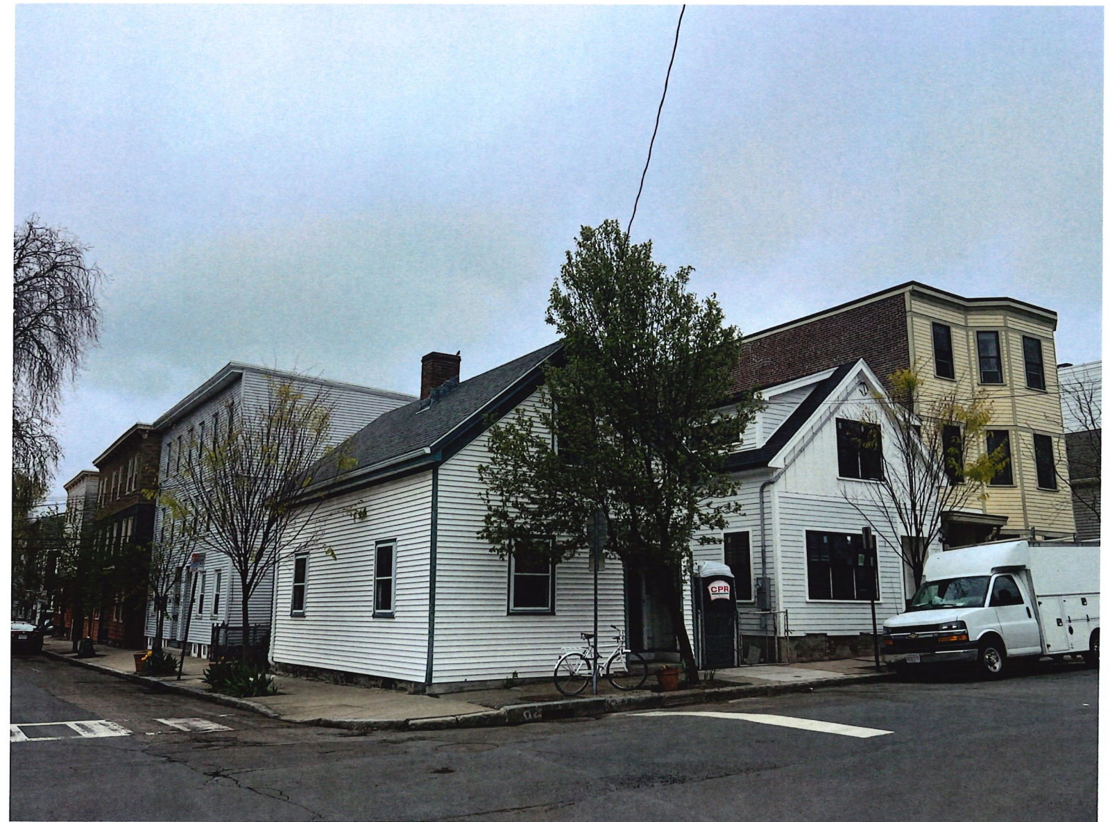
145 FIFTH STREET EXISTING STREET VIEW
