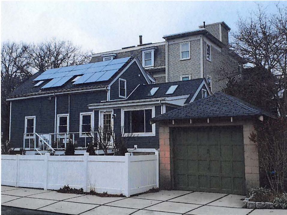
152 Pearl Street, VIEW FROM VALENTINE ST, Without railing
