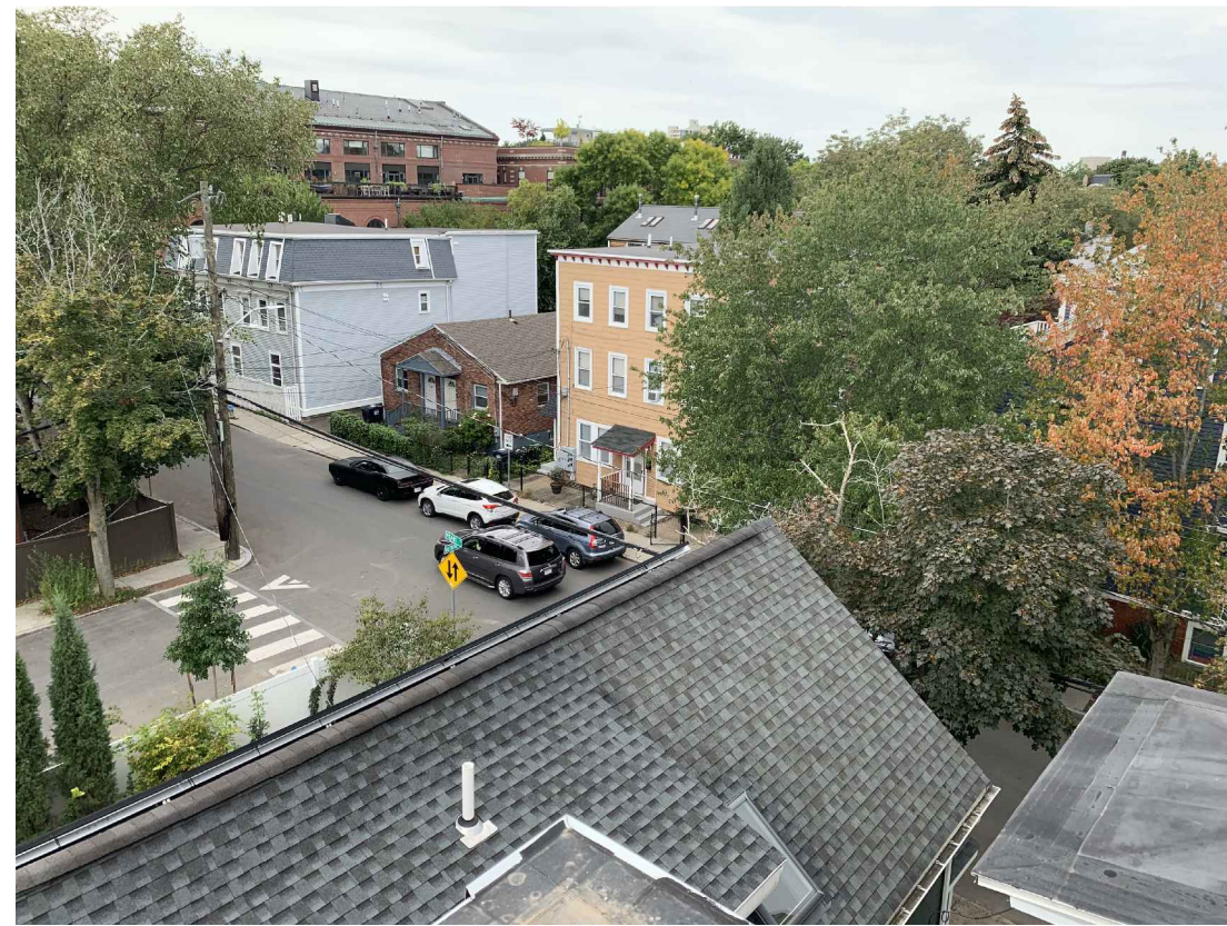
EXISTING ROOF VIEWS TOWARD VALENTINE AND PEARL STREET
