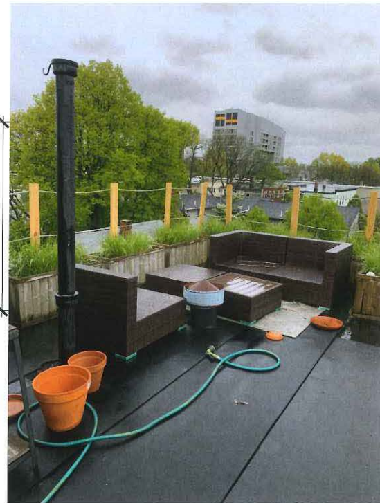
EXISTING ROOF DECK
