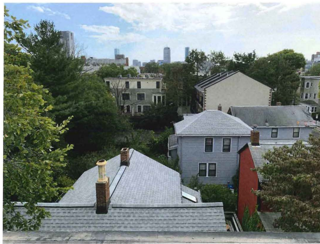
EXISTING ROOF VIEW TOWARD REAR
