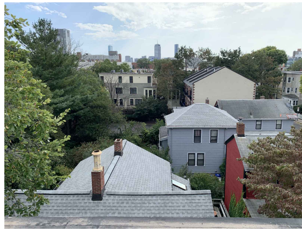
EXISTING ROOF VIEW TOWARD REAR
