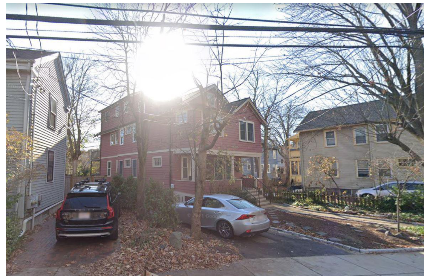
HOUSE DIRECTLY TO THE LEFT WITH SIMILAR THIRD FLOOR ADDITION
