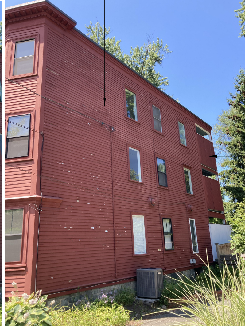
North (Right) Facade
