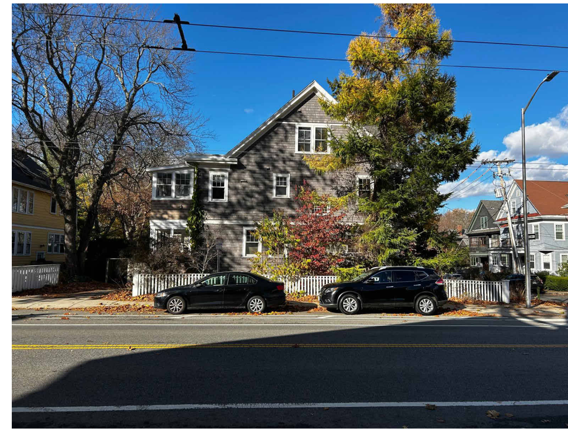
View of the south elevation, looking north from Huron Ave
