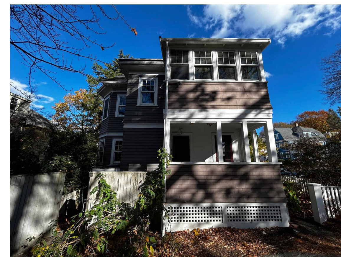
View of west elevation, looking east from the driveway
