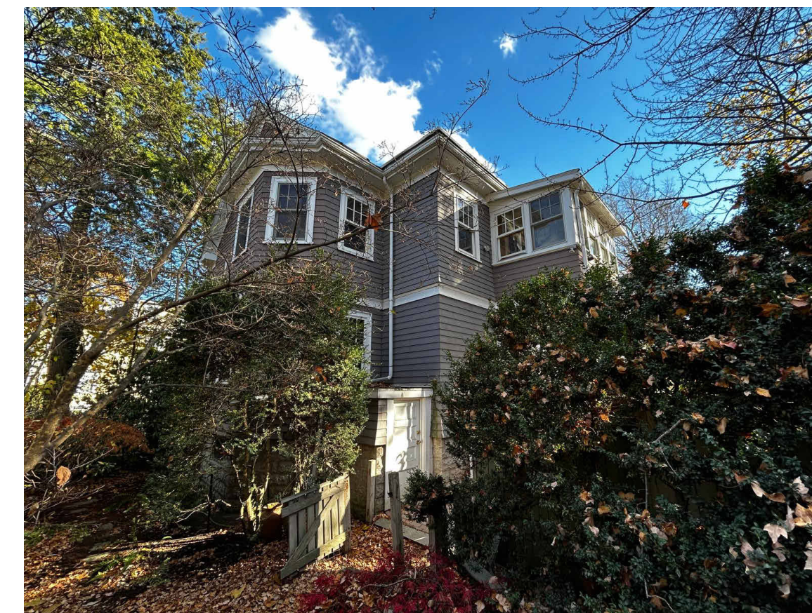
View looking southeast from the yard
