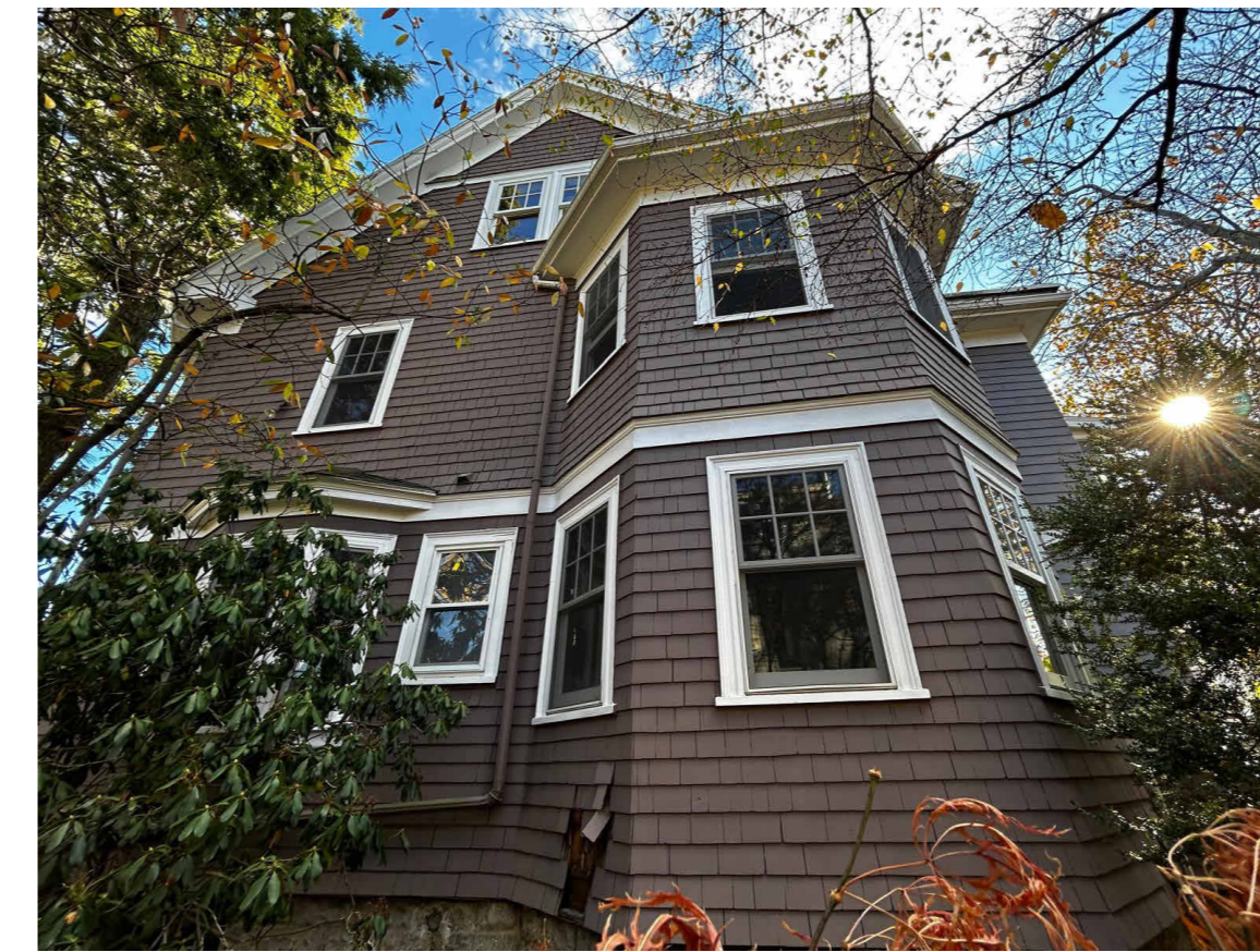
View of the north elevation, looking south from the yard
