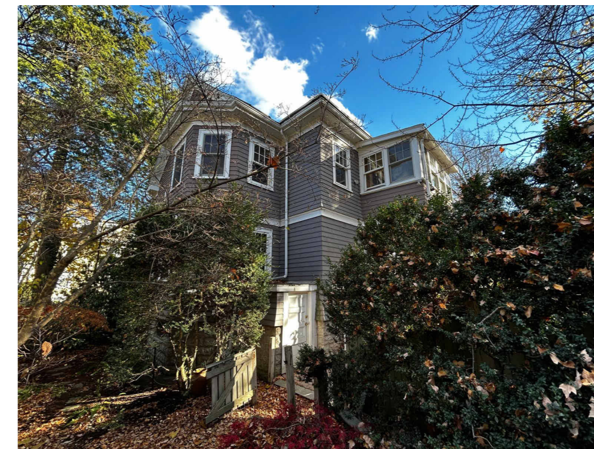
View looking southeast from the yard
