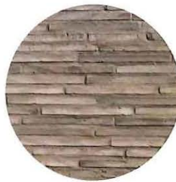
LONG MASONRY AT STREET LEVEL
