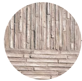
MASONRY SOLDIER COURSE AT HEADER
