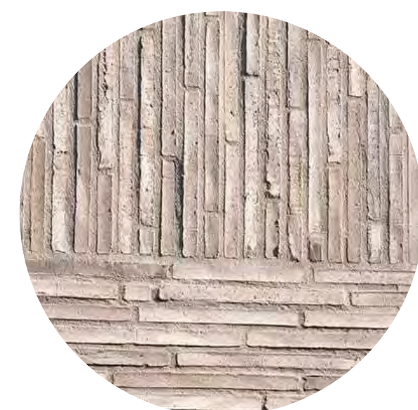
MASONRY SOLDIER COURSE AT HEADER
