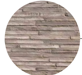
LONG MASONRY AT STREET LEVEL
