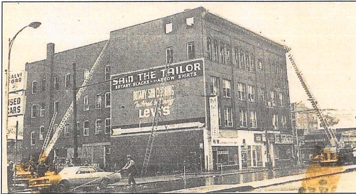
I.O.O.F. Building formerly located at 2072 Massachusetts Avenue, depicted during the 1968 fire which led to its demolition ( Cambridge Chronicle ).
