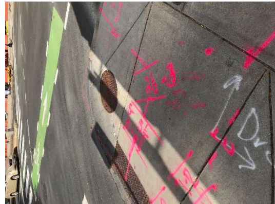
Manhole located on the corner of Walden and Mass Ave, enters the vault at 5-5.5 feet with multiple lines running to adjacent handholes and vaults 2-3 feet from the surface and 1-2 feet.
