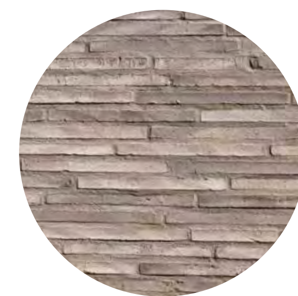
LONG MASONRY AT STREET LEVEL
