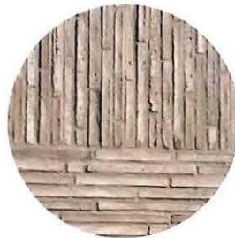
MASONRY SOLDIER COURSE AT HEADER
