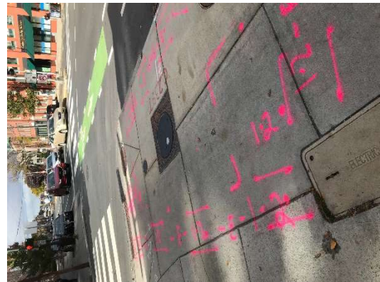
Electrical handhole located on the bottom right, potential signal or site lighting controls – electrical was being feed from a black transformer located on the sidewalk.
