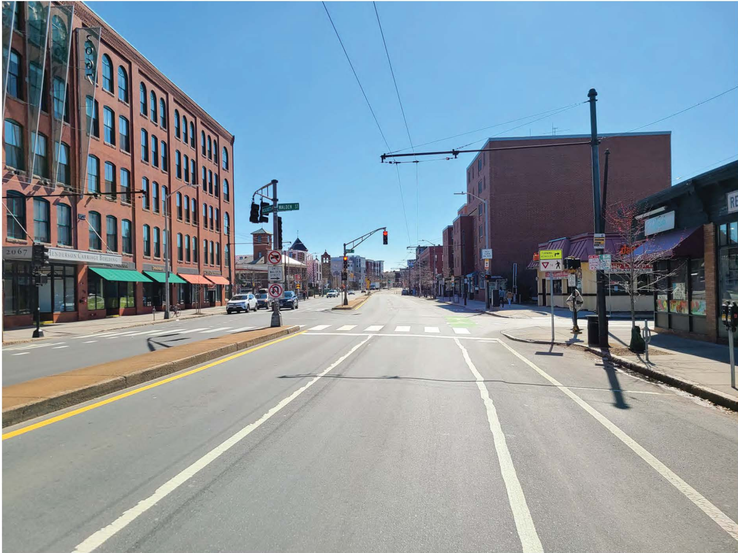
View on Massachusetts Avenue Looking South-East
