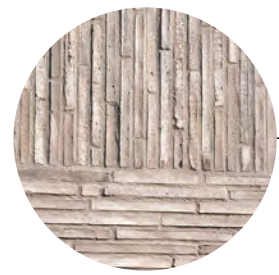
MASONRY SOLDIER COURSE AT HEADER
