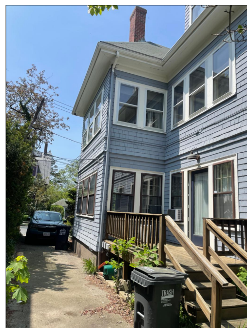
EXISTING VIEW OF SE CORNER
