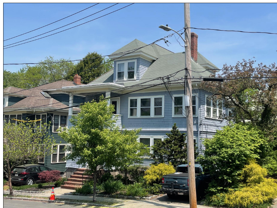
EXISTING VIEW OF SW CORNER
