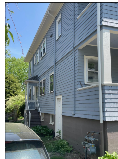
EXISTING VIEW OF NORTH FACADE
