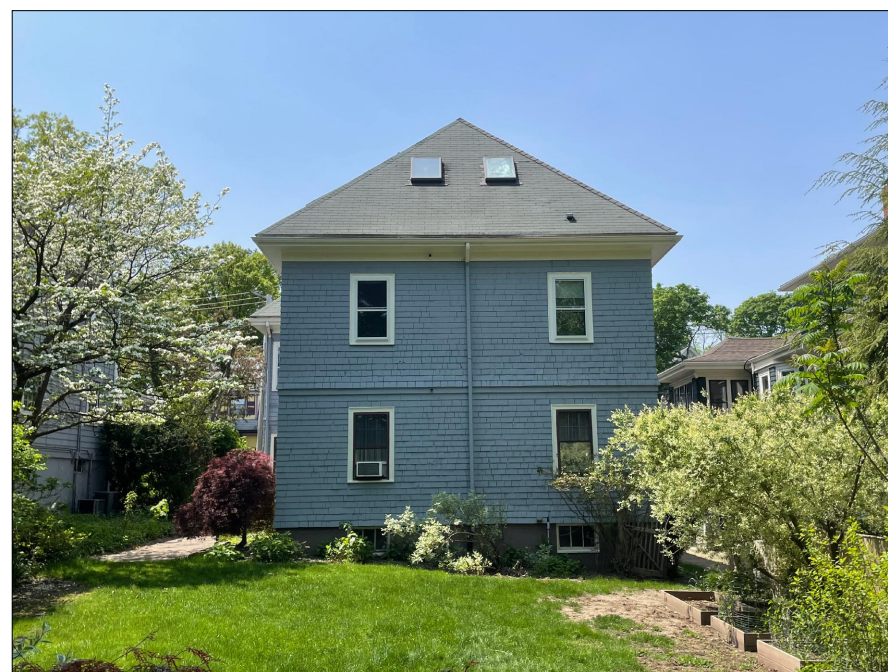
EXISTING VIEW OF EAST/REAR FACADE
