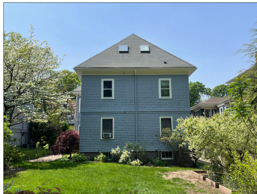
EXISTING VIEW OF EAST/REAR FACADE
