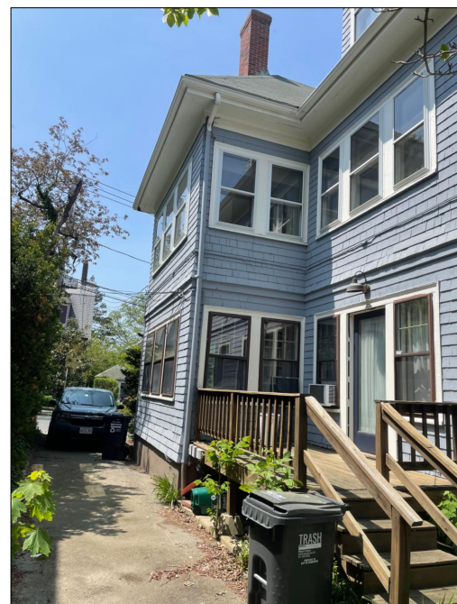
EXISTING VIEW OF SE CORNER
