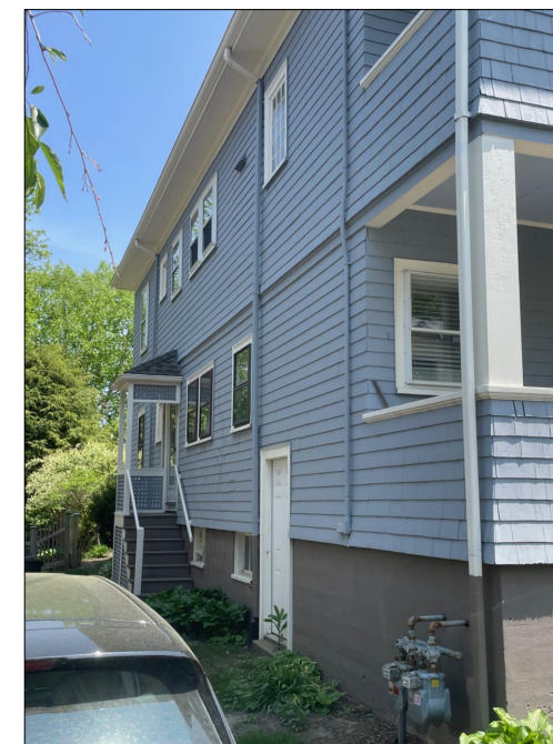
EXISTING VIEW OF NORTH FACADE
