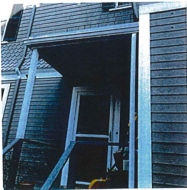
EXISTING CONDITION PHOTOS 25 BREWSTER STREET
