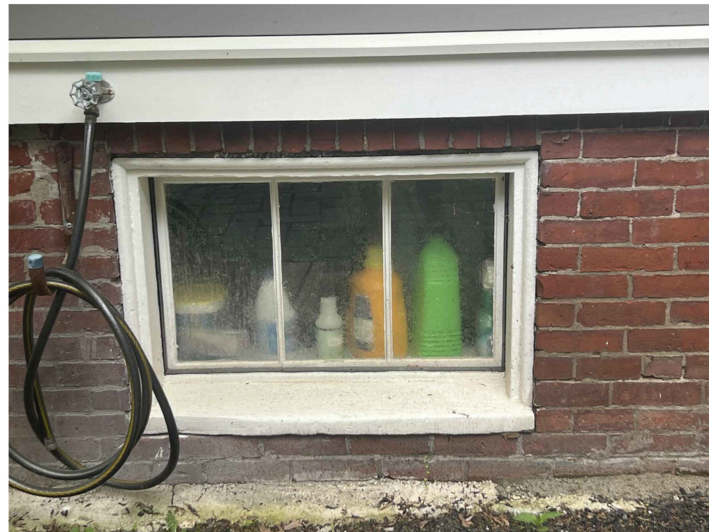
EXISTING WINDOW #1 TO BE ENLARGED AS PART OF NEW WINDOW WELL
