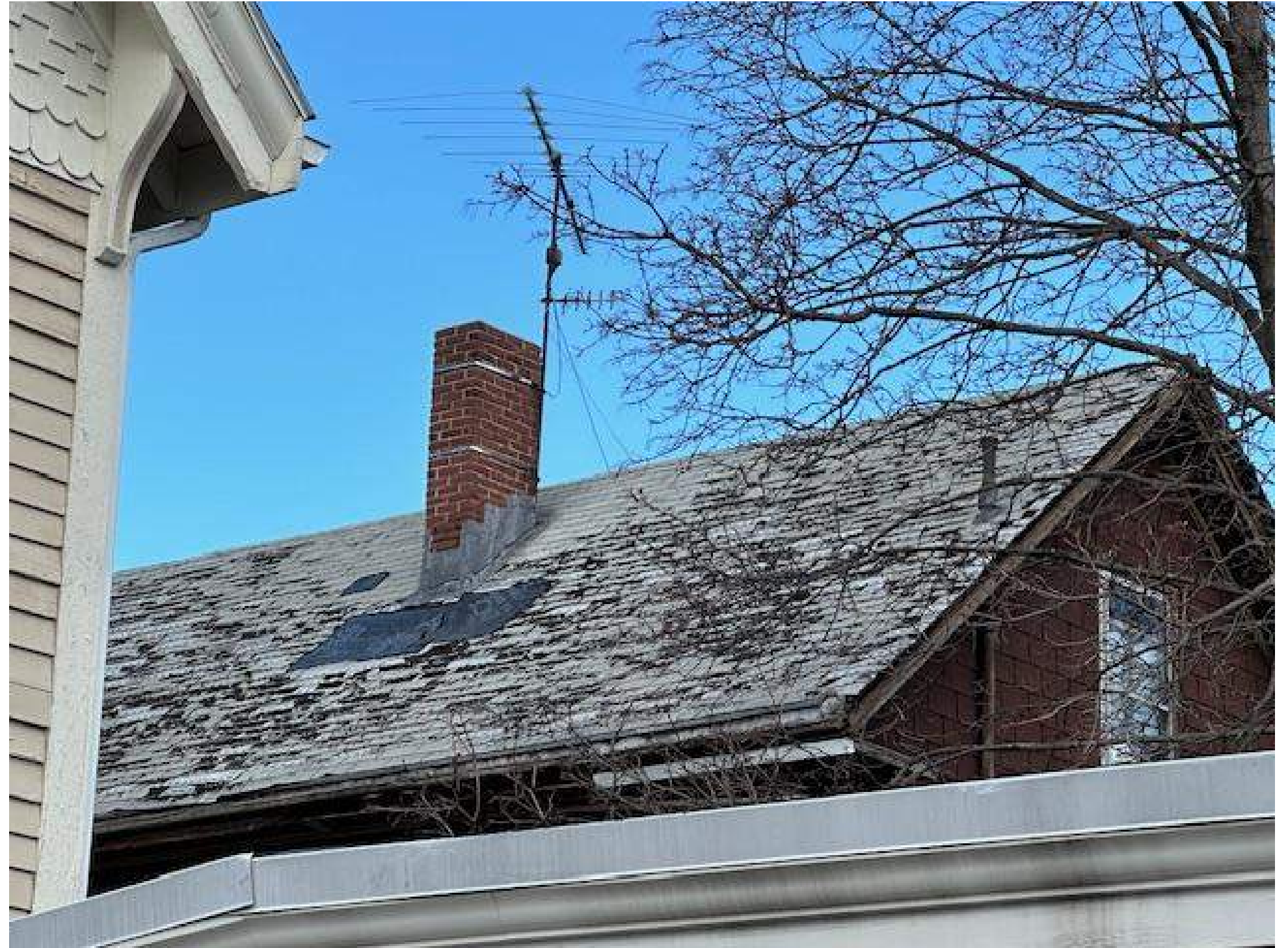
DETERIORATED ROOF
