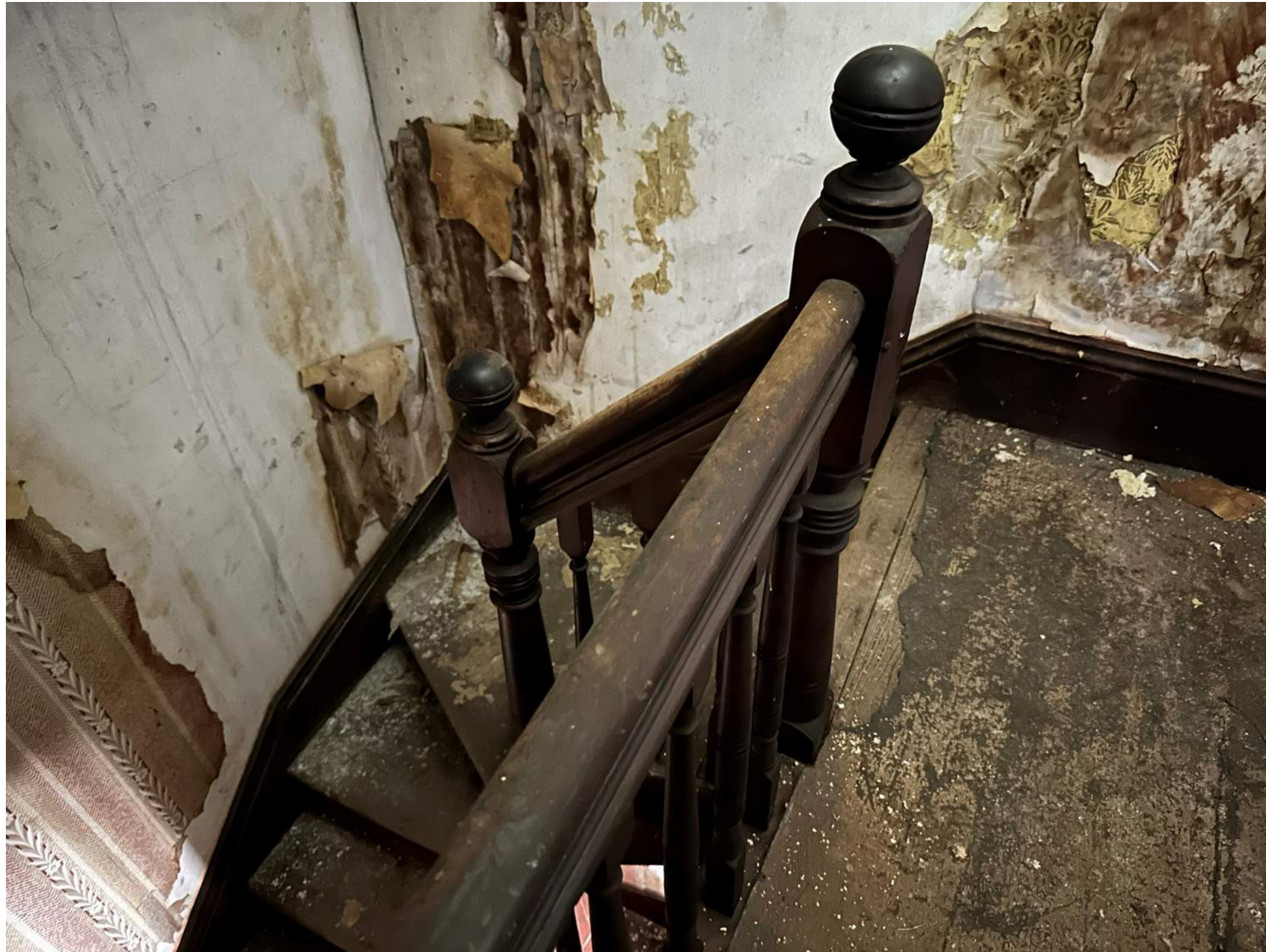
NOT TO CODE STAIR, WINDERS, RAILING AND HEAD HEIGHT
