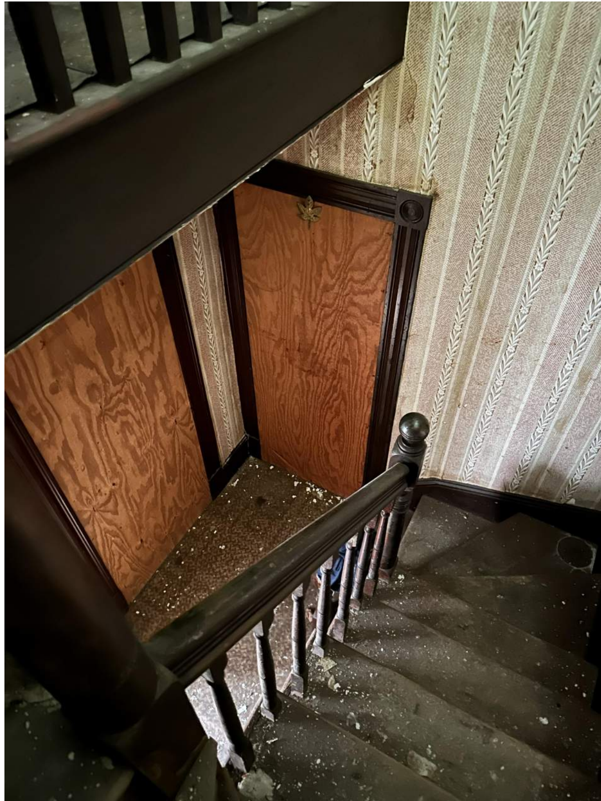
NOT TO CODE STAIR, WINDERS, RAILING AND HEAD HEIGHT
