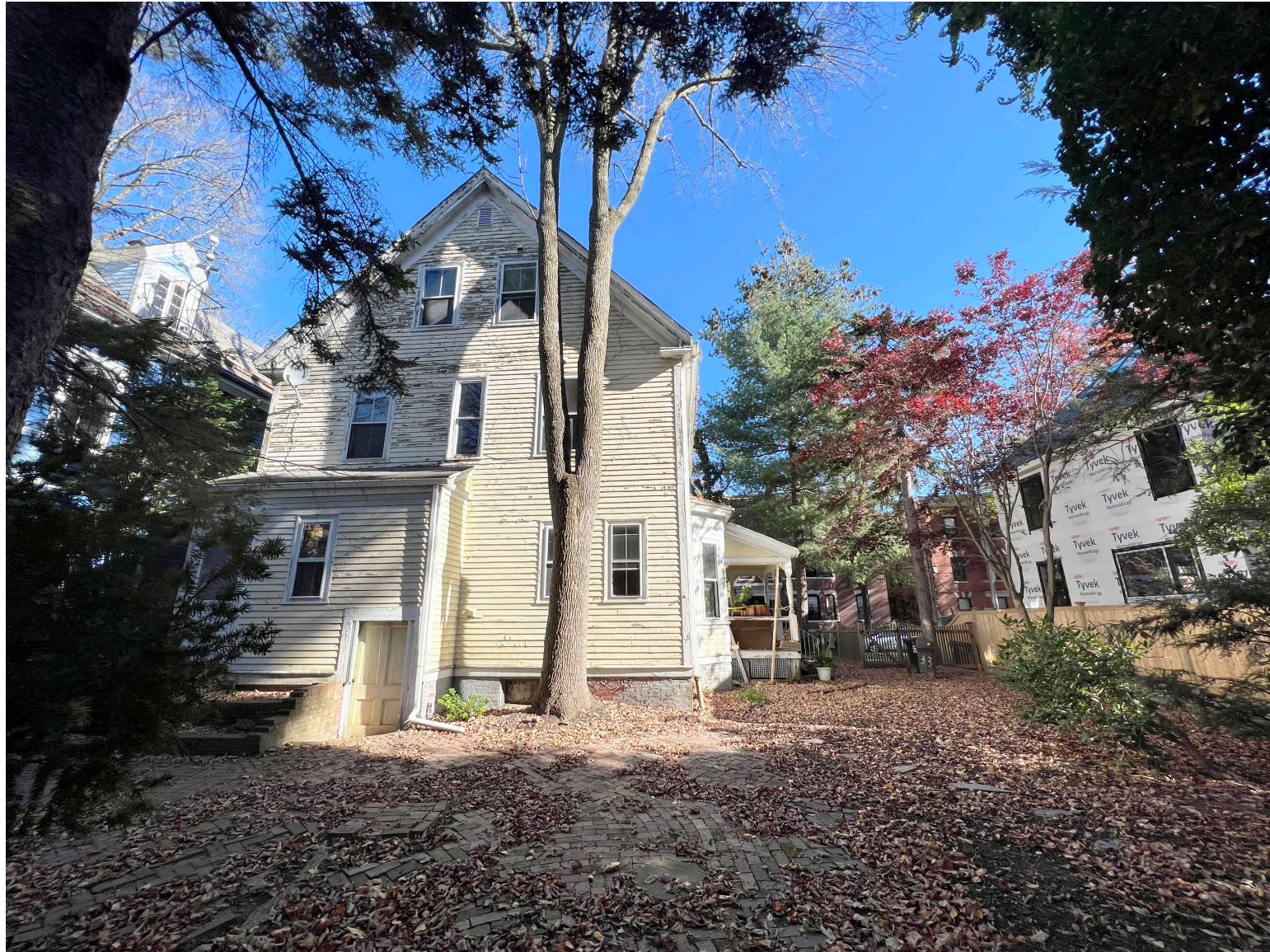
33 HURLBUT EXISTNG VIEW FROM REAR
