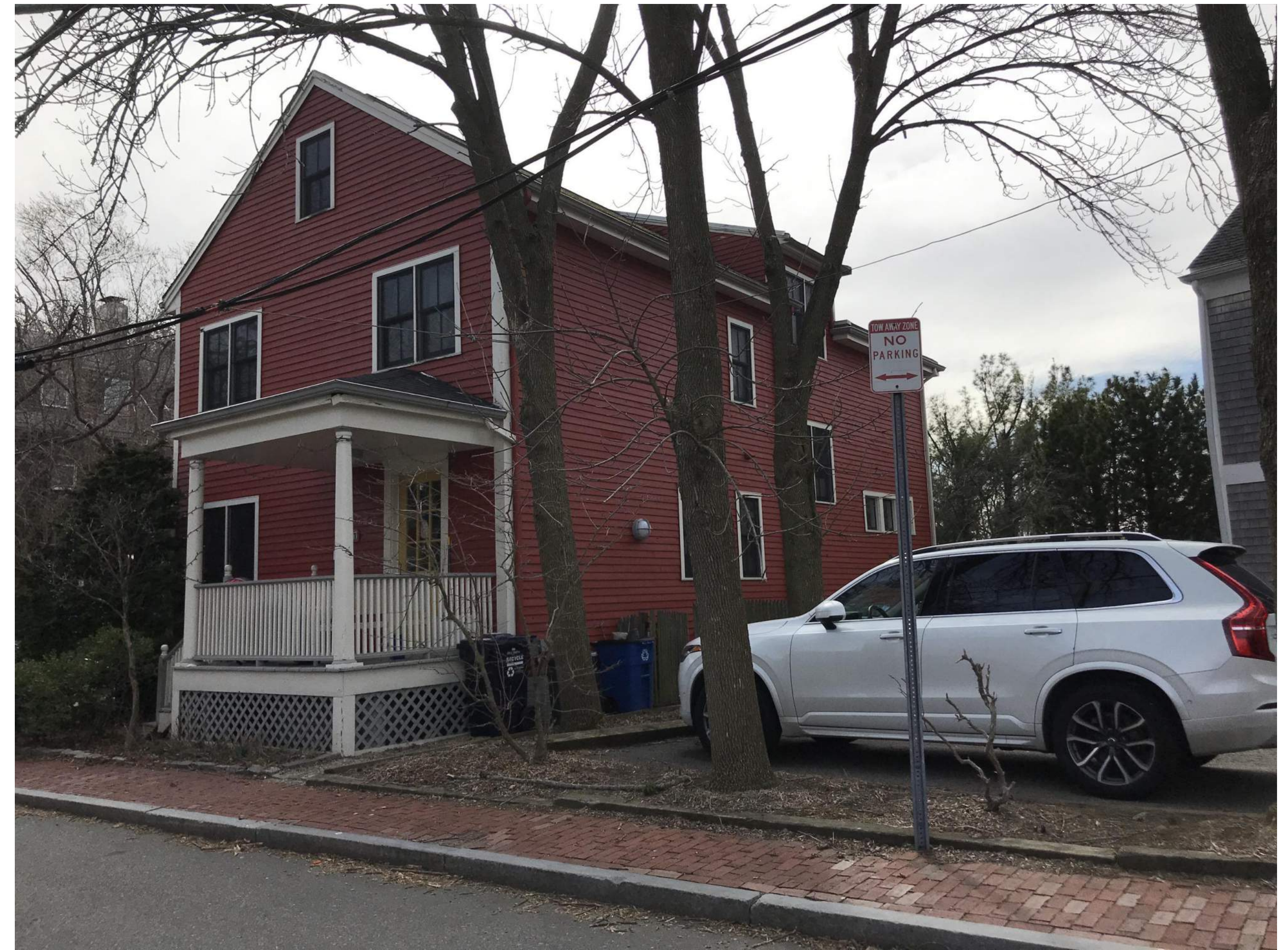
EXISTING FRONT OF HOUSE
