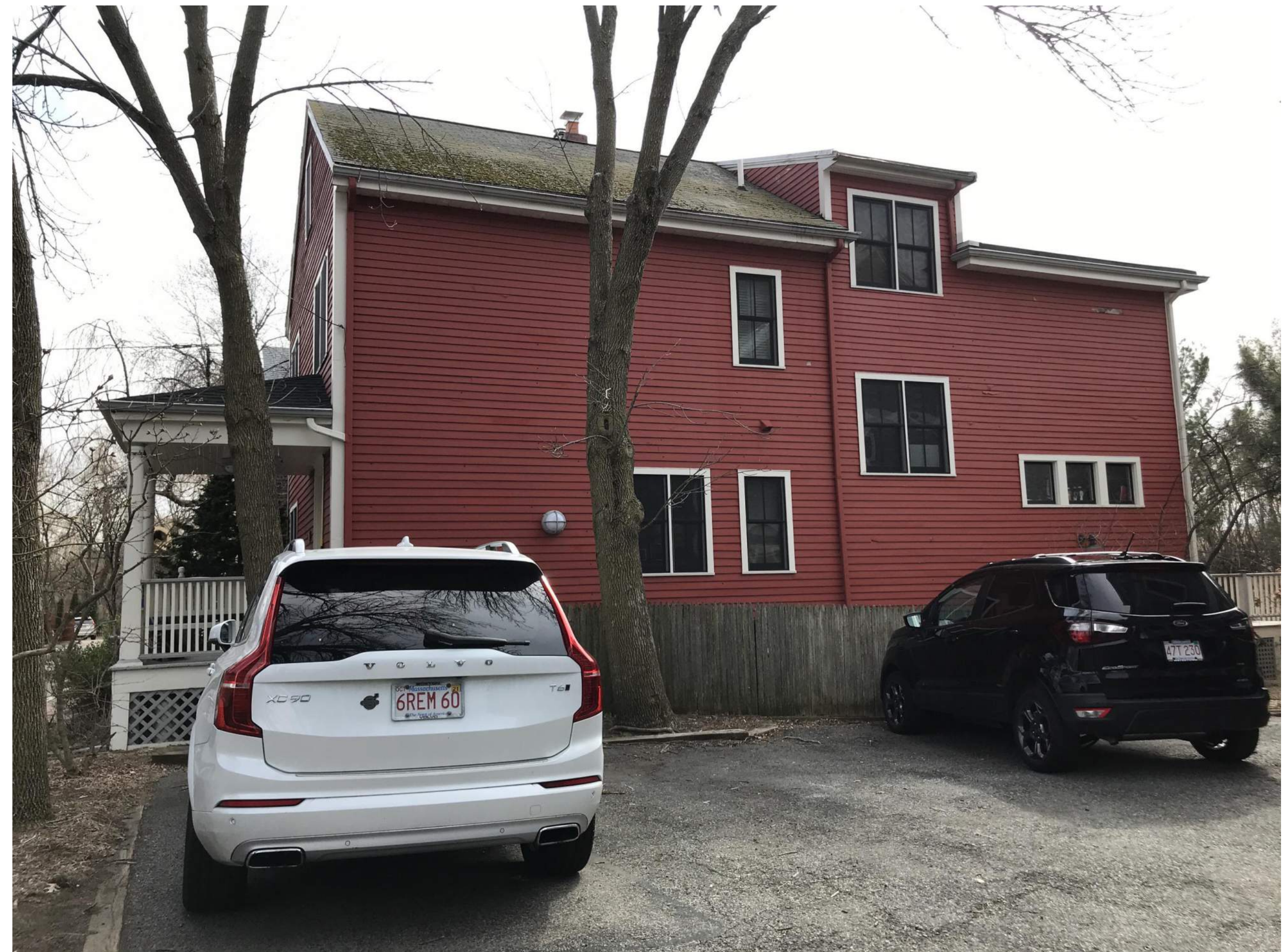
EXISTING RIGHT SIDE OF HOUSE
