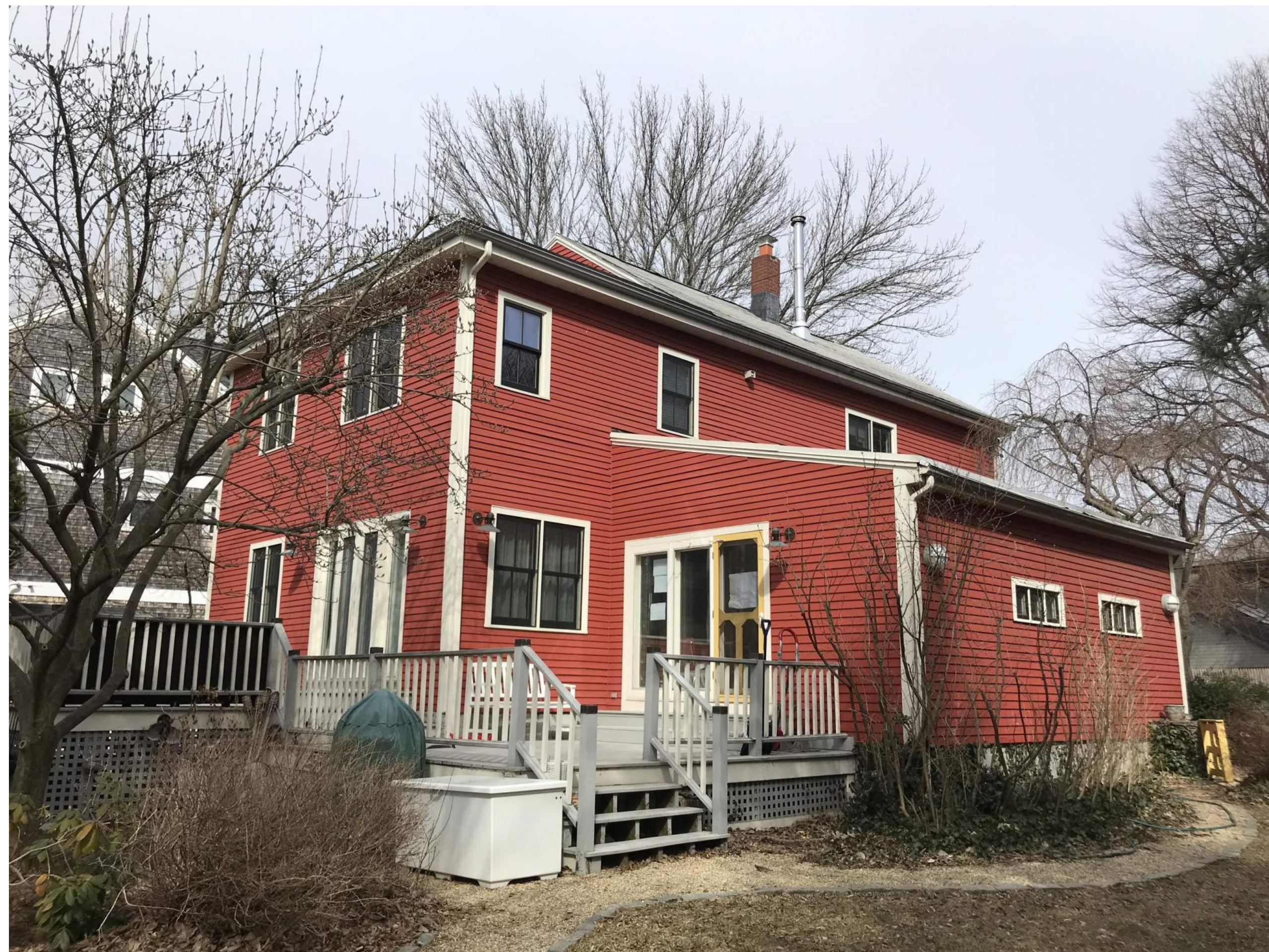
EXISTING REAR OF HOUSE
