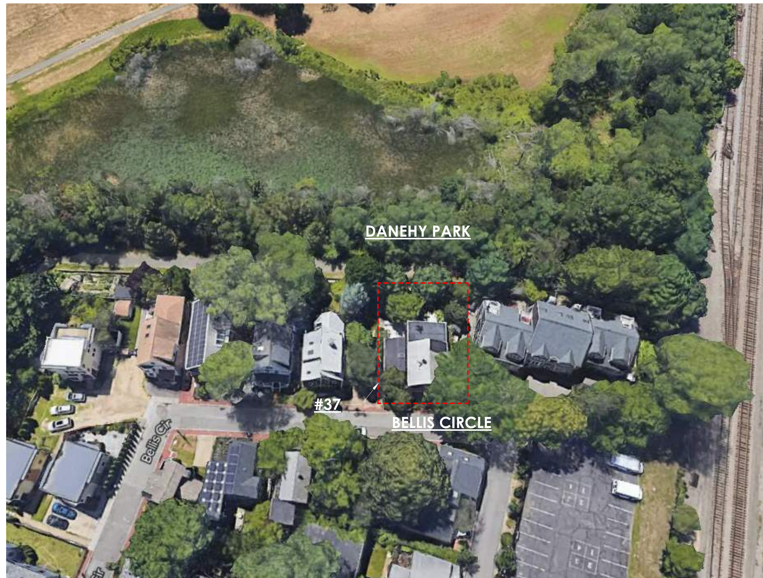
EXISTING AERIAL VIEW
