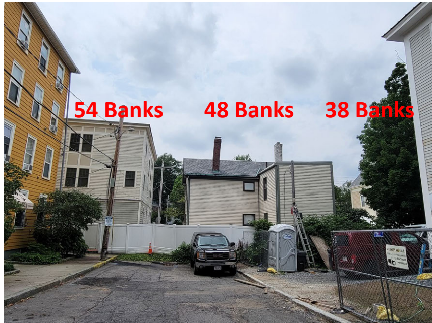
Green Street – West End View of project site from Green Street
