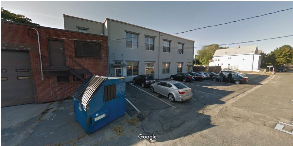
Photo 4: North East view of proposed trailer location
