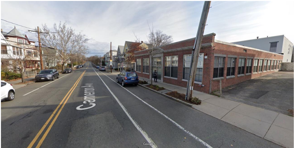
Photo 2: North West view of 38 Cameron Avenue
