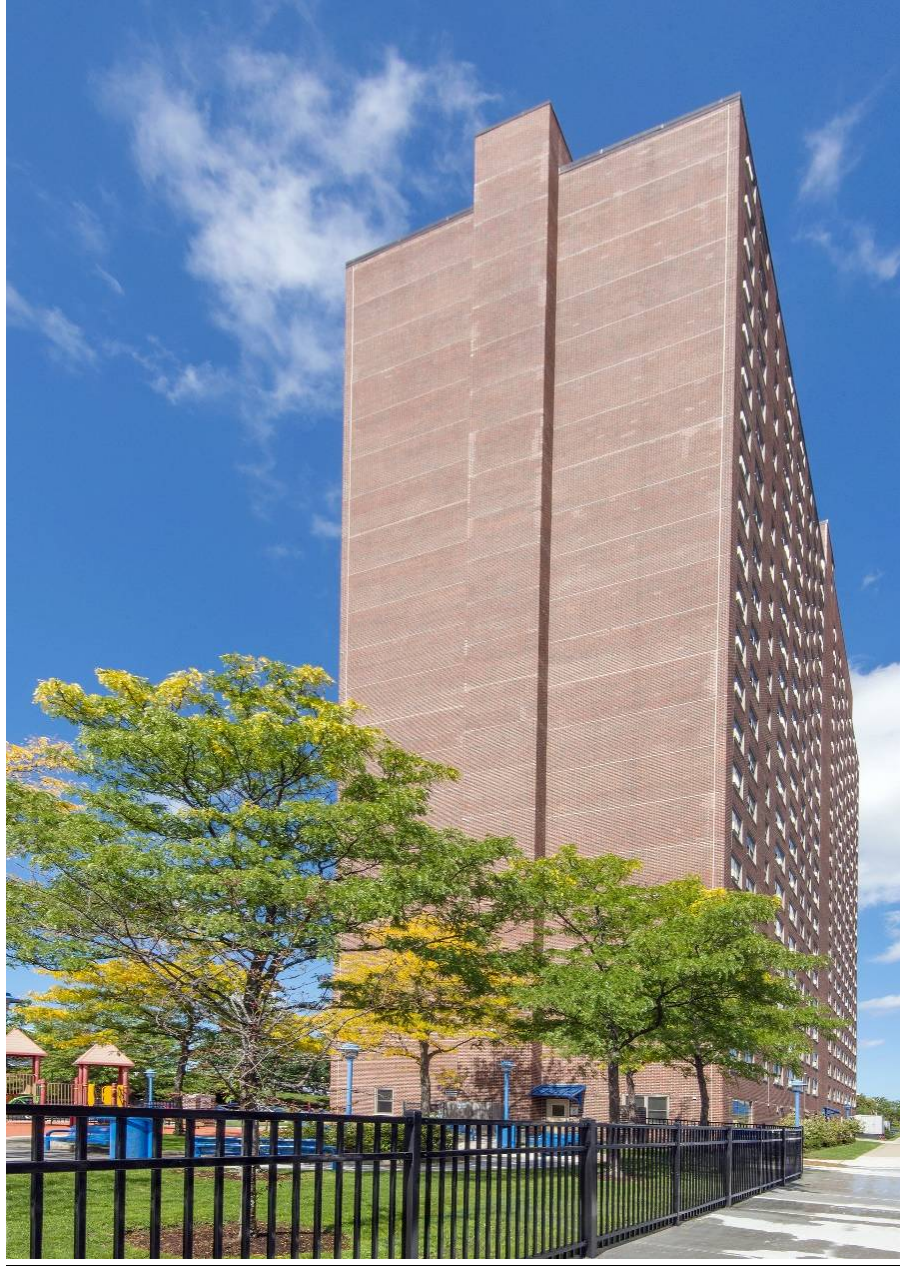
Existing building from Southeast
