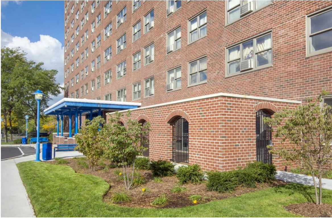
Existing Building Front Entry and Patio
