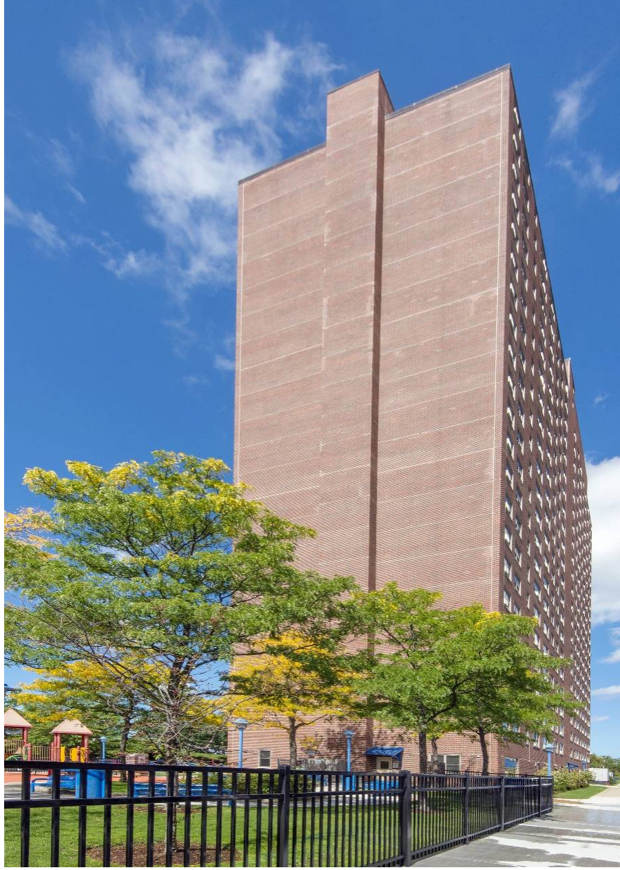
Existing building from Southeast
