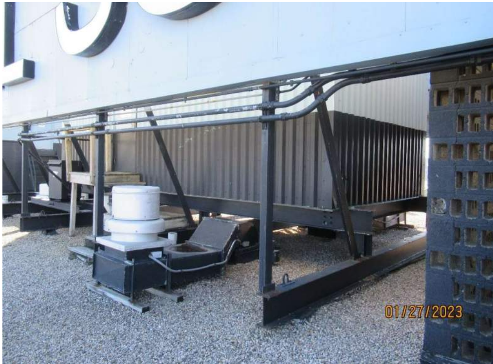
Photo 4: Sample photo illustrating the existing roof construction.
