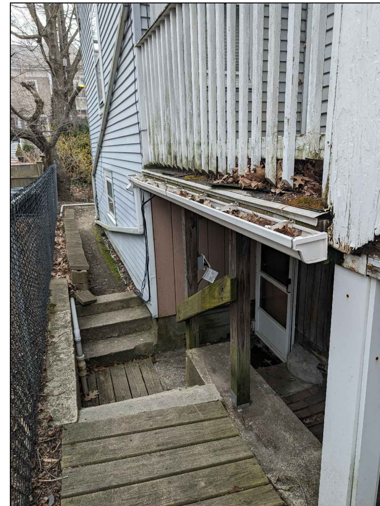
G View of Lower Unit Entry Door
