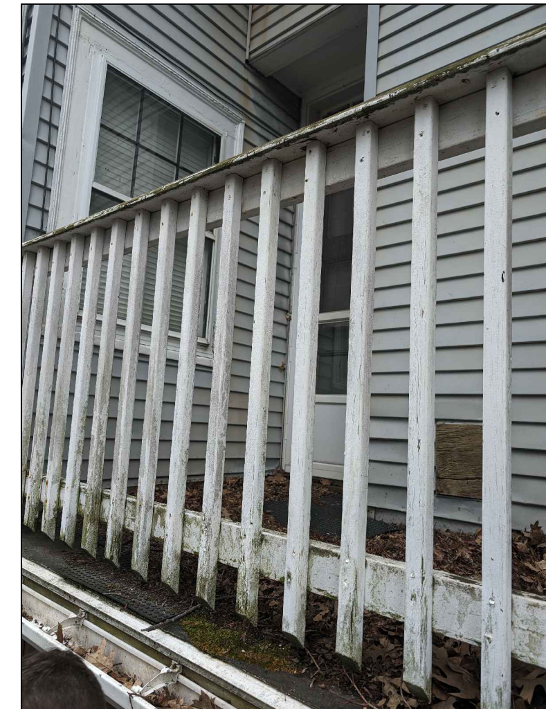
H Side View of First Floor Deck
