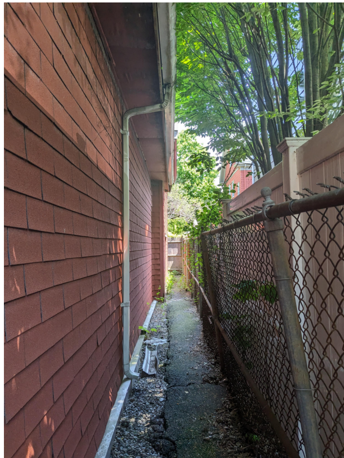
SITE PHOTO - BARN REAR
