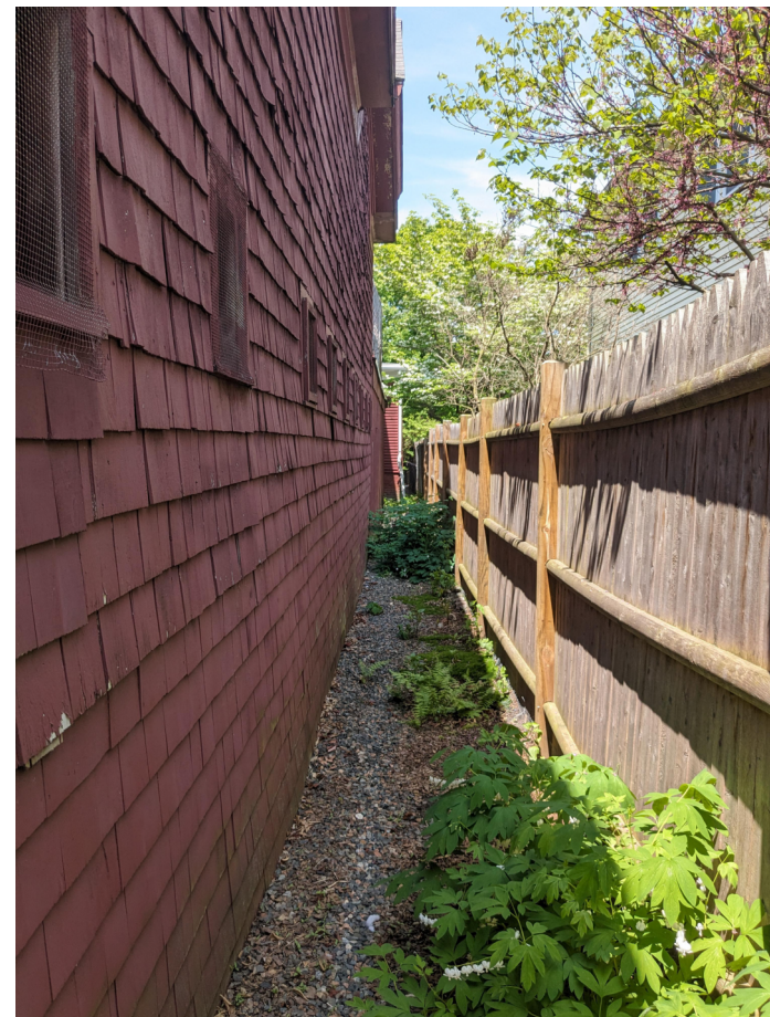
SITE PHOTO - BARN LEFT
