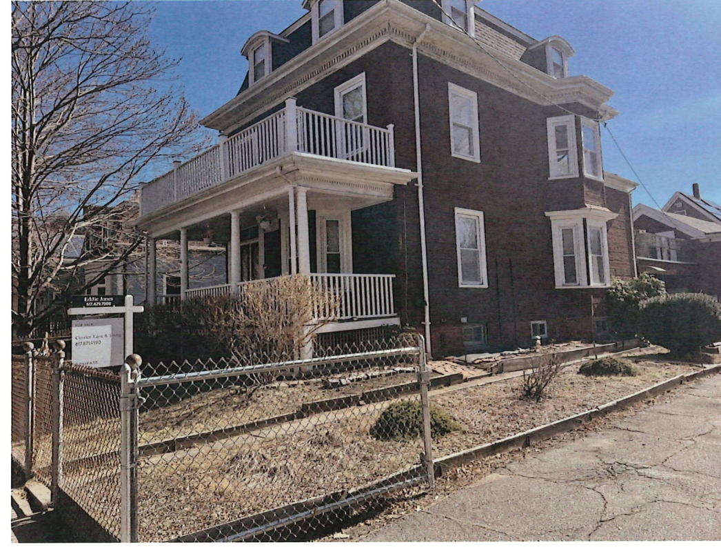
SITE PHOTO - VICINITY OF AREAWAY
