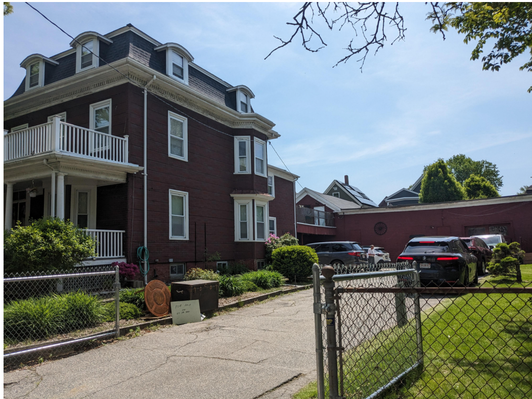
SITE PHOTO - SITE OVERVIEW
