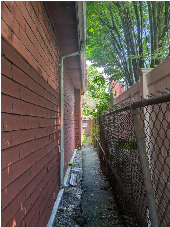
SITE PHOTO - BARN REAR
