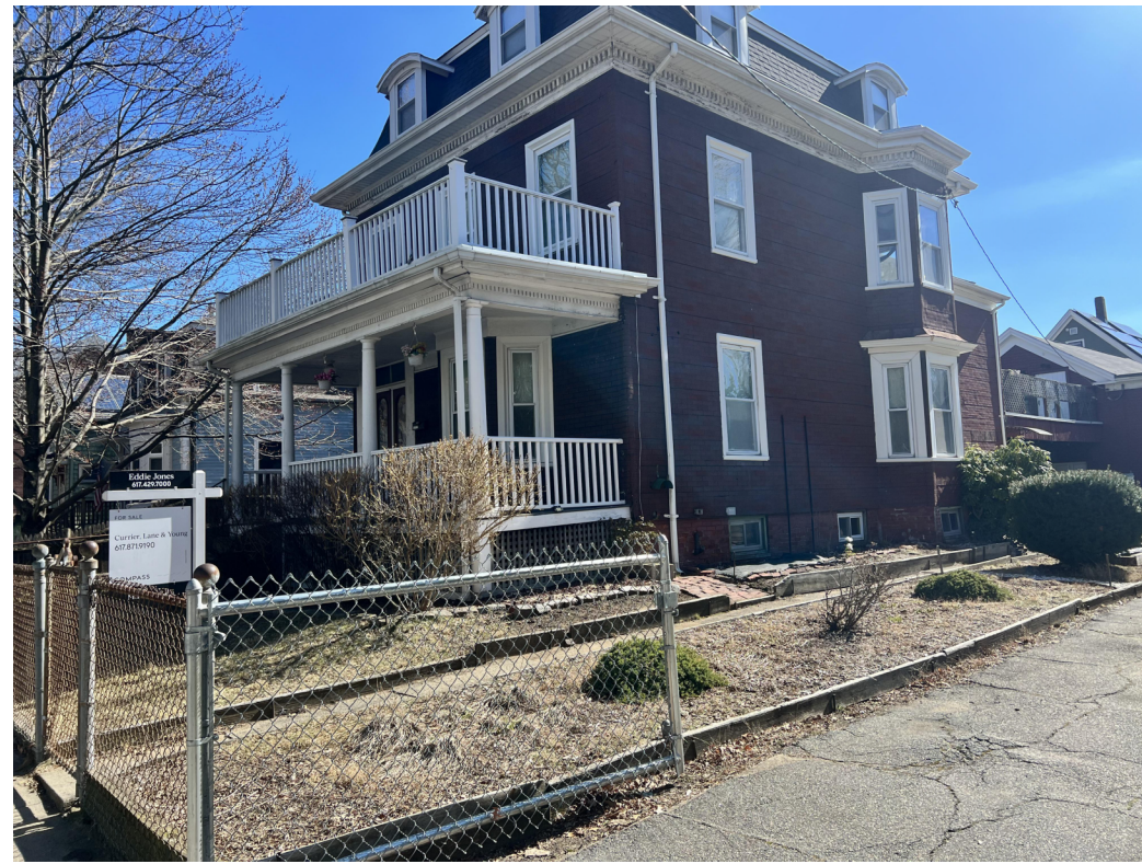
SITE PHOTO - VICINITY OF AREAWAY
